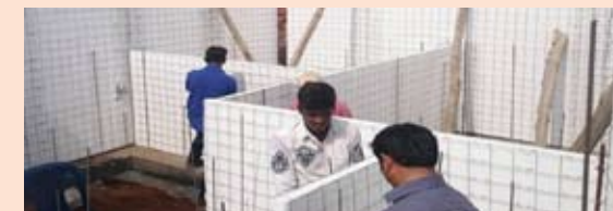
Houses being constructed by Govt. of Andhra Pradesh (using prefab technology)
