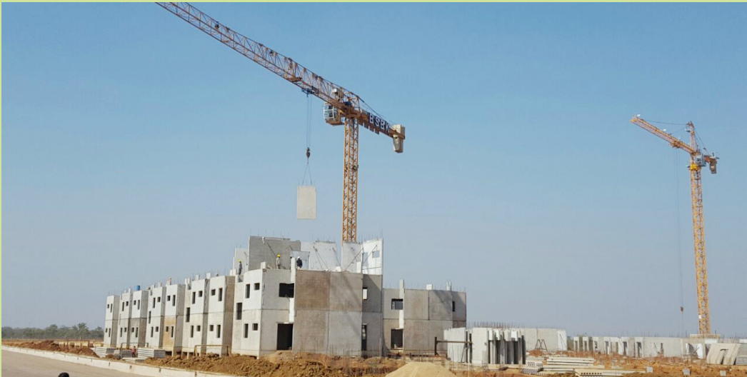
AHP under Construction Houses using pre-cast technology in Naya Raipur, Chhattisgarh
