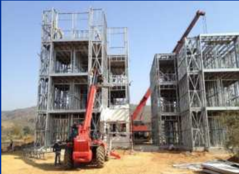
Cold-formed Steel Construction
