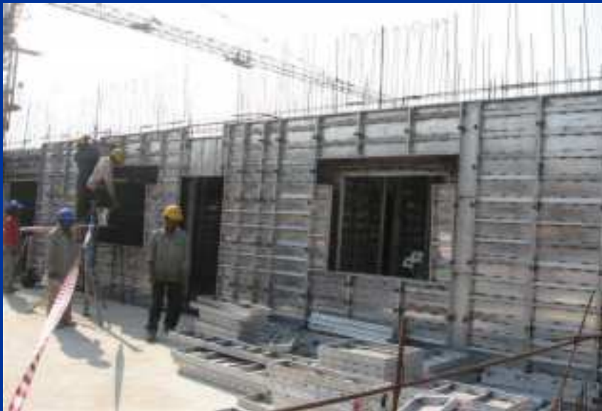
MIVAN formwork used for the construction of South City residential complex, Bangalore
