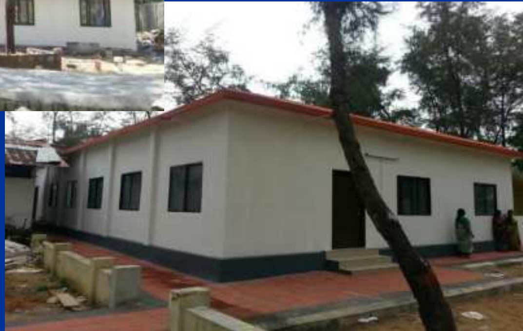
Canteen building (built-area – 1,600 sq.ft.)
