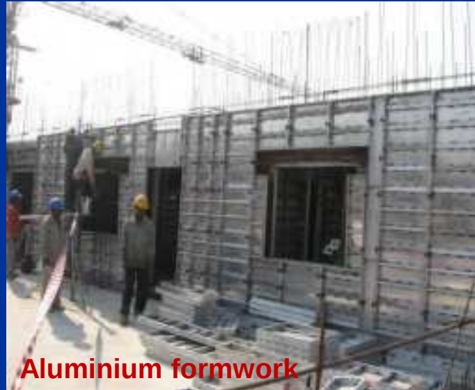
Large area formwork
