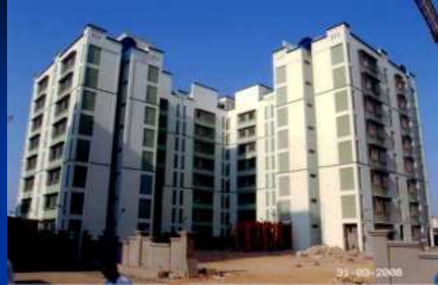
Light-weight Concrete Building
