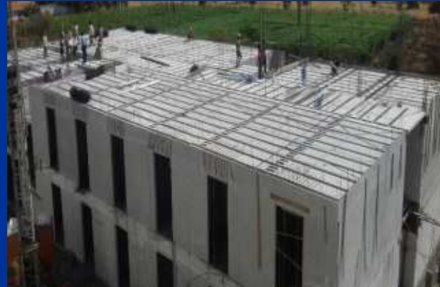
GFRG Building Construction
