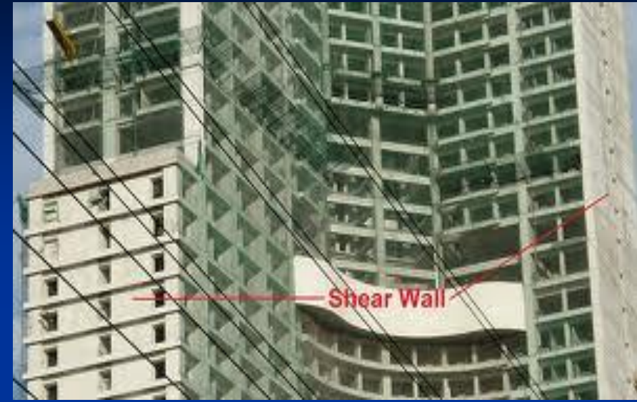
Shear Wall Building Construction
