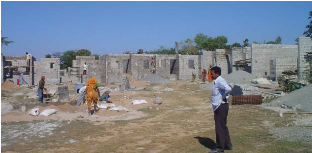
Demonstration Houses under VAMBAY being constructed by BMTPC at Bilaspur, Chhattisgarh
