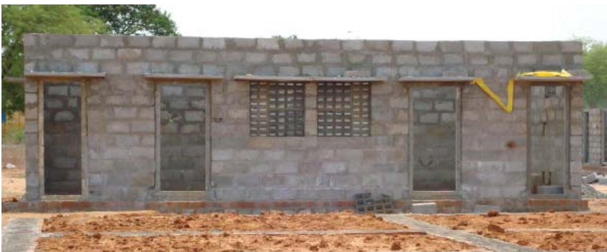
Demonstration Houses under VAMBAY being constructed by BMTPC at Trichi, Tamil Nadu
