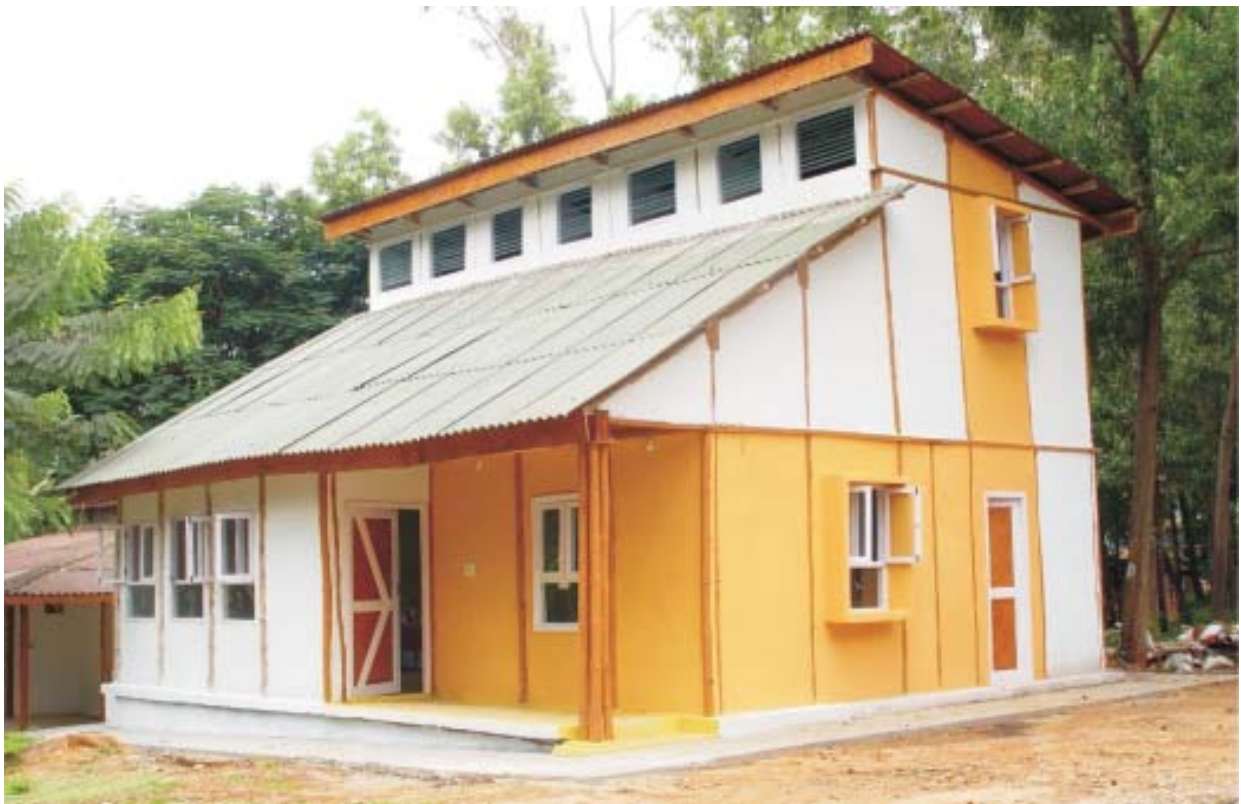
BMTPC developed a Technology for construction of two storey bamboo housing system at IPIRTI Bangalore.
