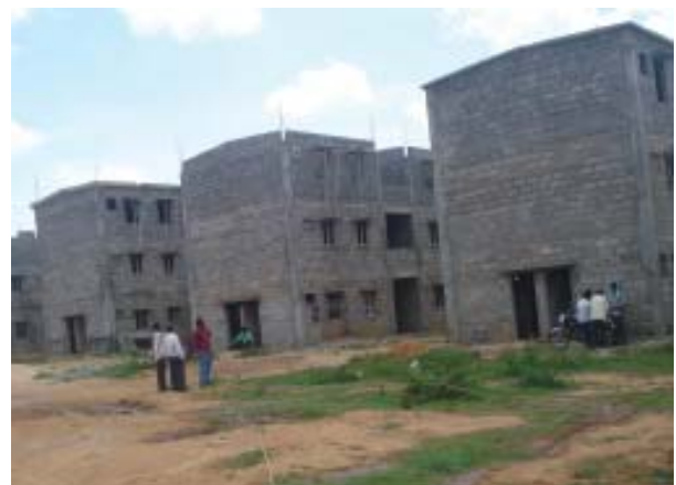
Demonstration Houses under VAMBAY being constructed by BMTPC at Kudalu, Karnataka
