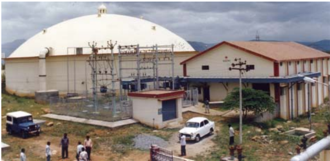
Provision of Piped Water Supply to Rural Habitations in Tamil Nadu (Phase V – 32.70 lakh litre capacity Ground Level Water Storage Reservoir with booster station at Kunjandiyur in Salem District, Tamil Nadu)
