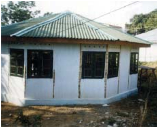
Construction of Demonstration Library Building using bamboo based technologies at Kolasib, Mizoram by BMTPC
