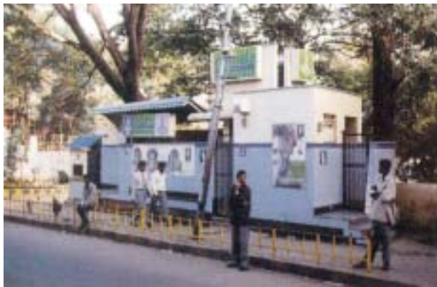
'Nirmala' – Pay and Use Toilet Complex, Bangalore, Karnataka by Bangalore Mahanagara Palike (Scheme No. 17739)
