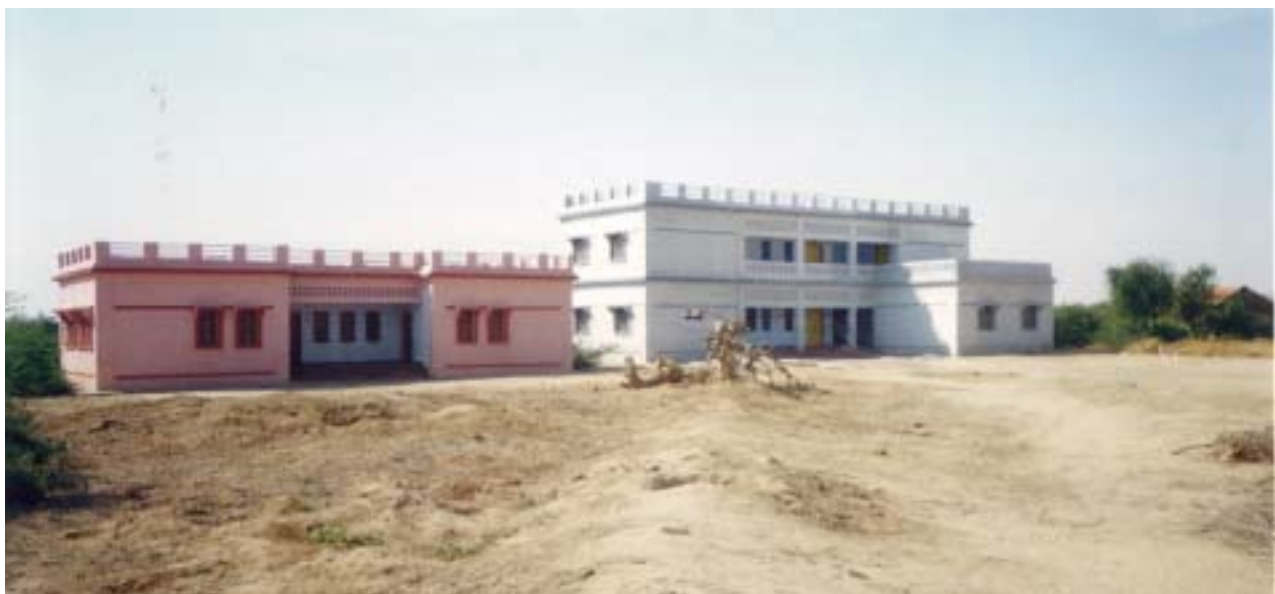
Primary Schools (PS3 & PS6) at Gedi Village, Rapar, Kutch, Gujarat constructed under MPLAD works.
