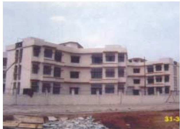
Housing for Urban Poor at Borsojai, Assam
