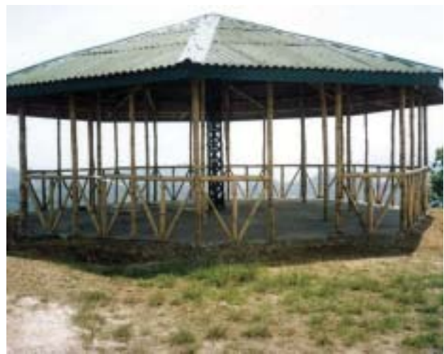
Construction of Demonstration Picnic Hut using bamboo based technologies at Aizawl, Mizoram by BMTPC
