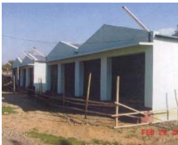
Slum Upgradation - Shopping Stalls at Iroisemba, Imphal, Manipur
