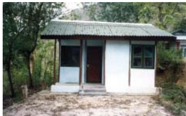
Construction of Demonstration Small House using bamboo based technologies at Sairang, Aizawl, Mizoram by BMTPC
