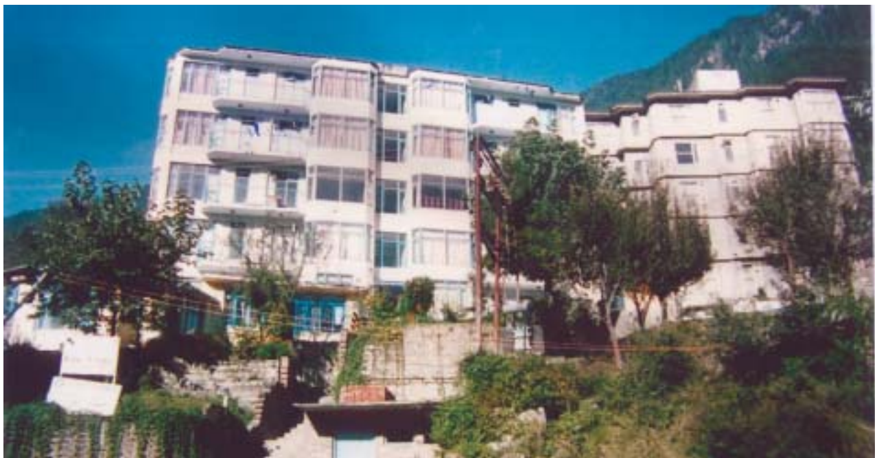
A Cooperative Housing Project at Manali (Himachal Pradesh)
