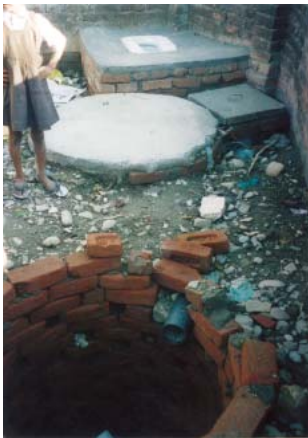
ILCS Unit under construction at Udham Singh Nagar Distt., Uttranchal in ILCS Scheme in 39 Towns Scheme No. 17597 – Agency SUDA, Dehradun
