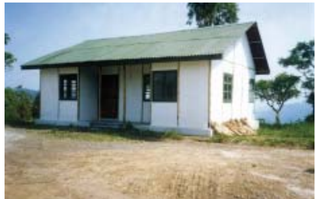
Construction of Demonstration Large House using bamboo based technologies at Aizawl, Mizoram by BMTPC
