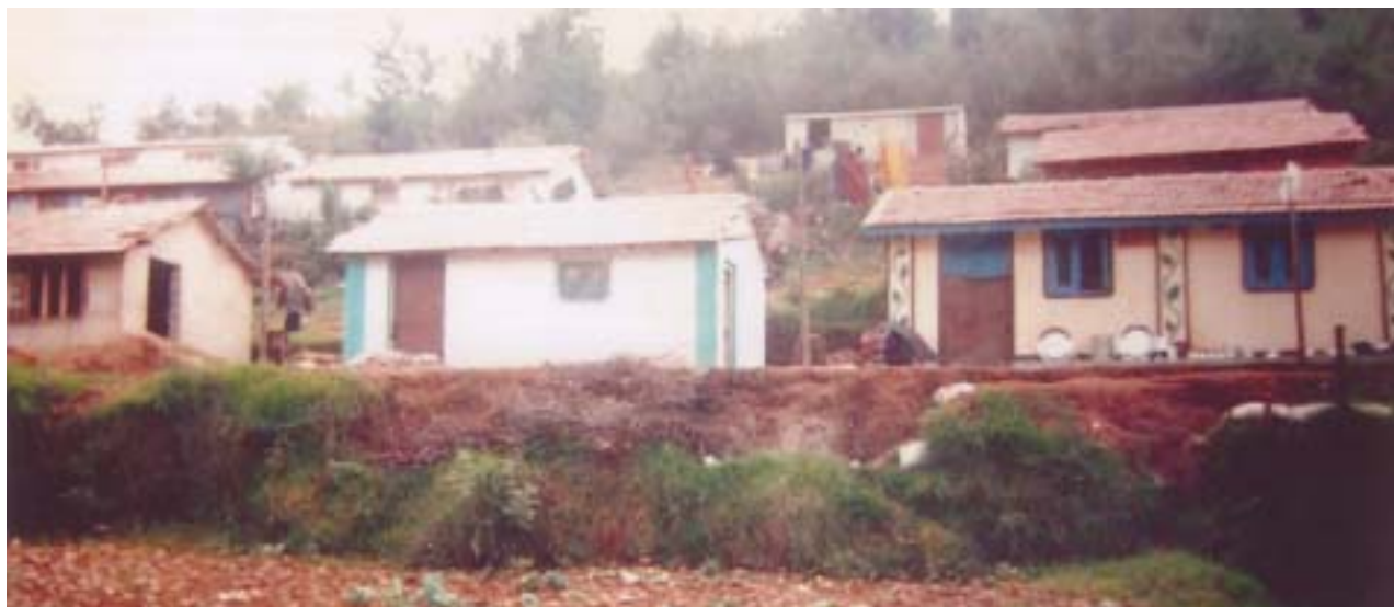
A Low Cost Cooperative Housing Project at Adikaratty (Tamil Nadu)
