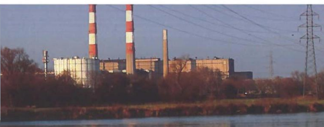
Power Plant, Koradi
