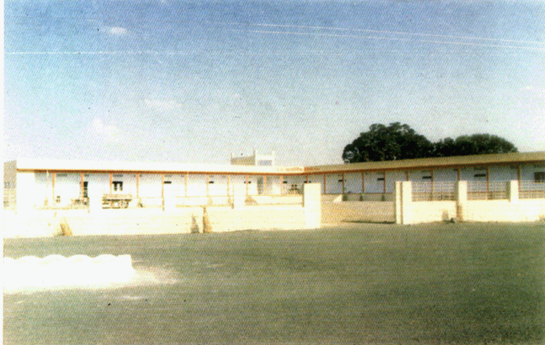
Construction of Primary School under Model Basti Scheme by Jalgaon Municipal Council
