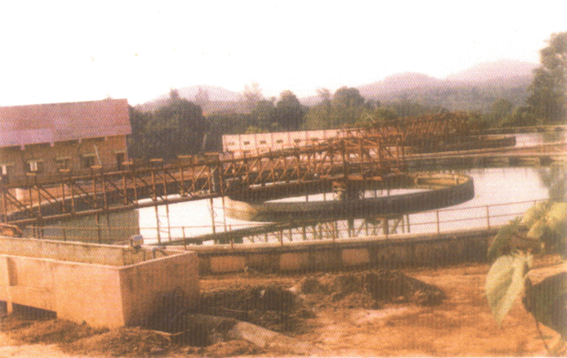
Trivandrum Water Supply Scheme, Water Treatment Plant. Agency: Kerala Water Authority
