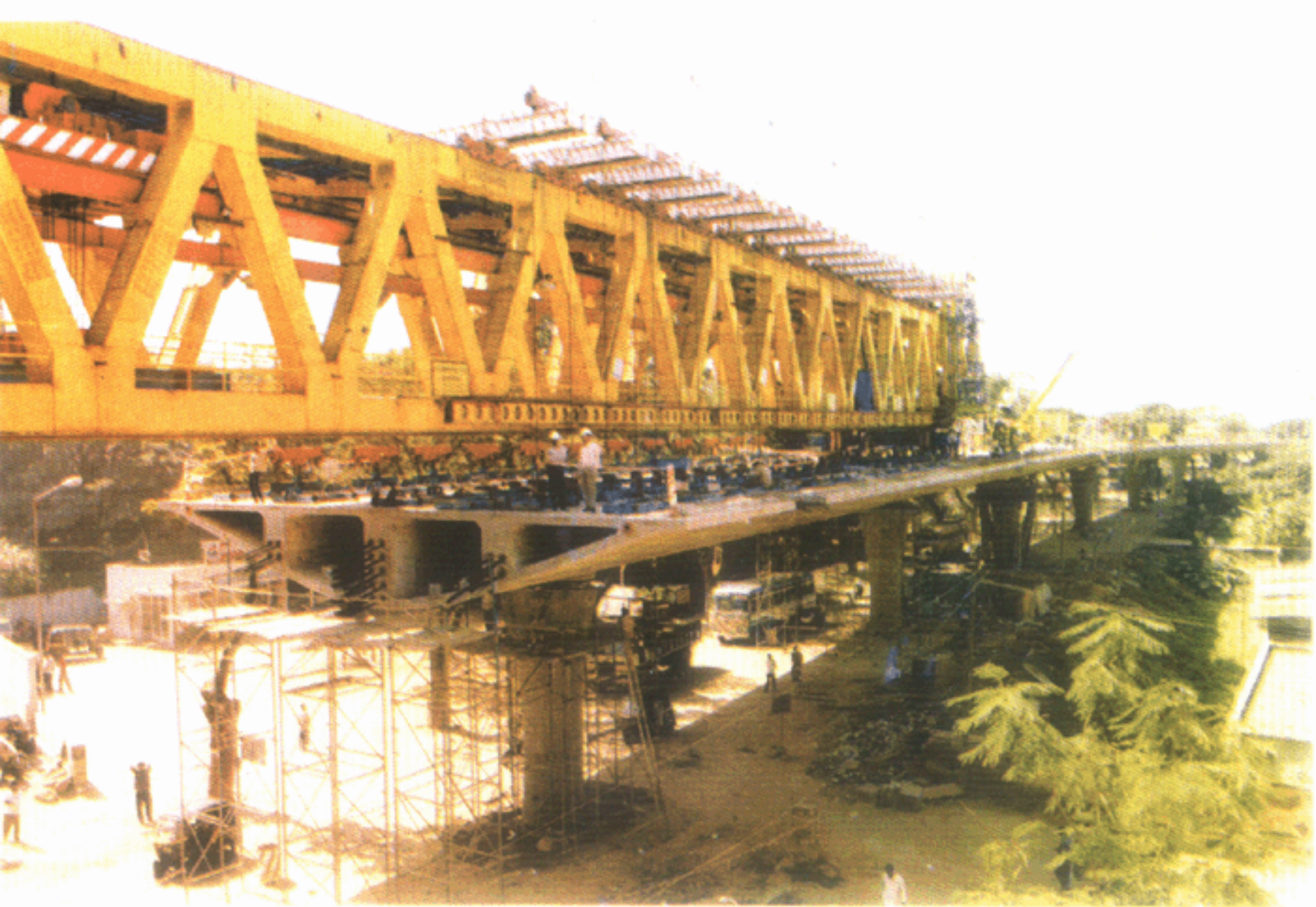
Construction of Sirsi Circle Flyover under Mega City Scheme
