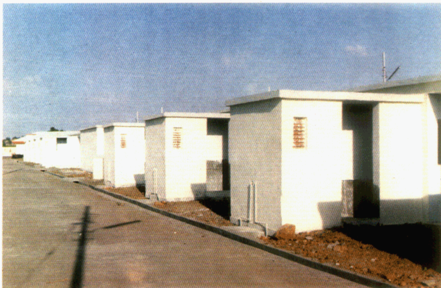
Construction of LIG Housing at Pimorala Jalgaon, Jalgaon Municipal Council
