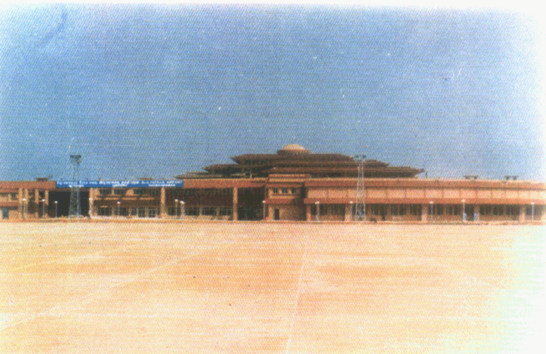
View of New Terminal of Biju Patnaik Airport at Bhubaneswar (Orissa)
