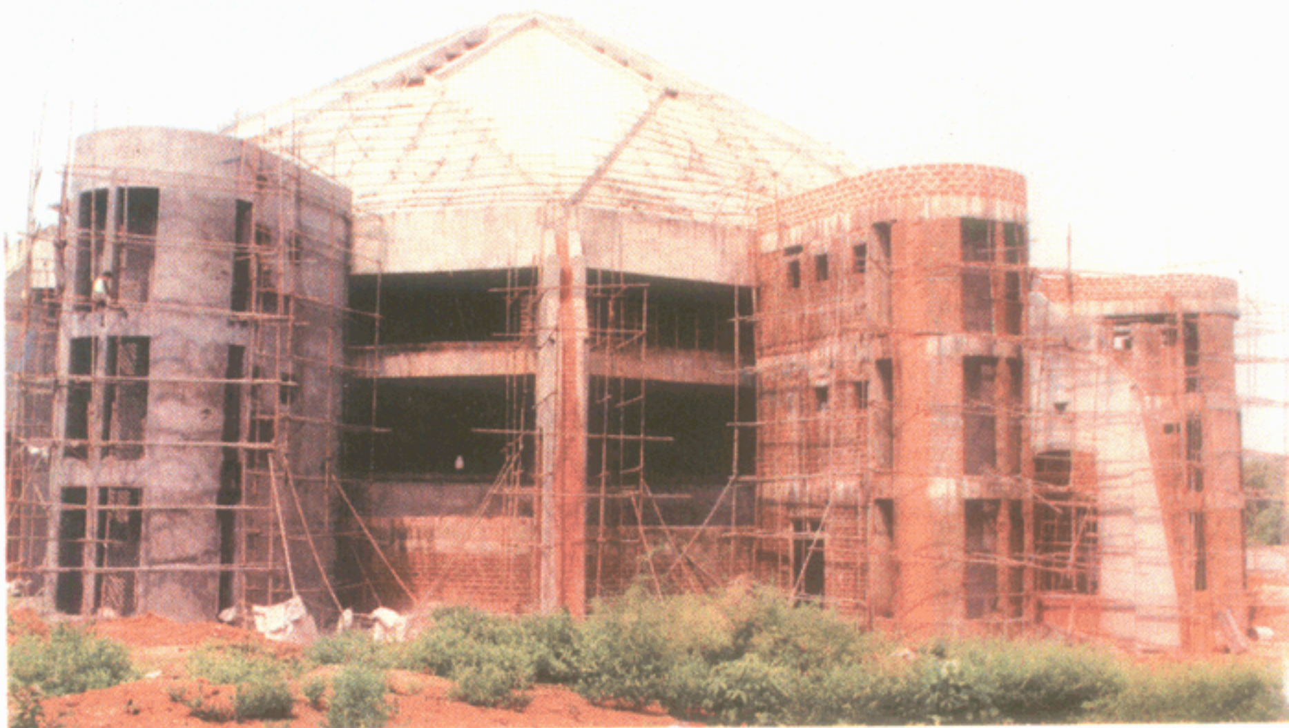
Construction of Legislative Assembly at Panaji, Goa with Loan Assistance from HUDCO
