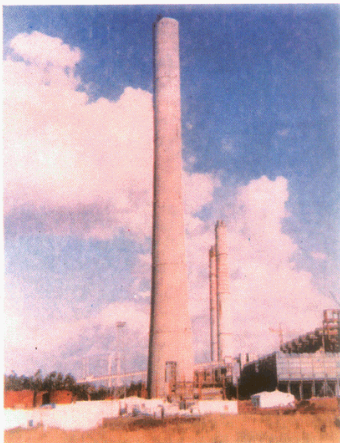
275 m High RCC Chimney for 2 x 500 MW Vindhyachal Super Thermal Power Project Stage-II at Vindhyachal for NTPC—NBCC
