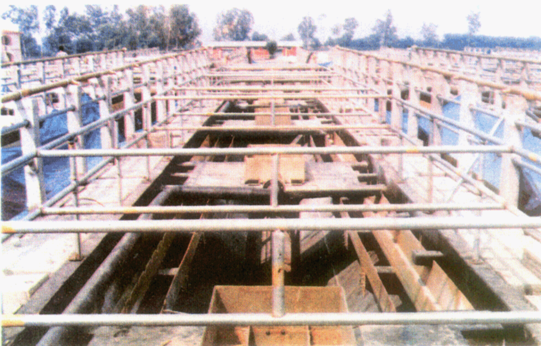
45 MLD Sewage Treatment Plant using Un Aerobic Sludge Blanket Technology under Yamuna Action Plan, provided for Haryana PWD.
