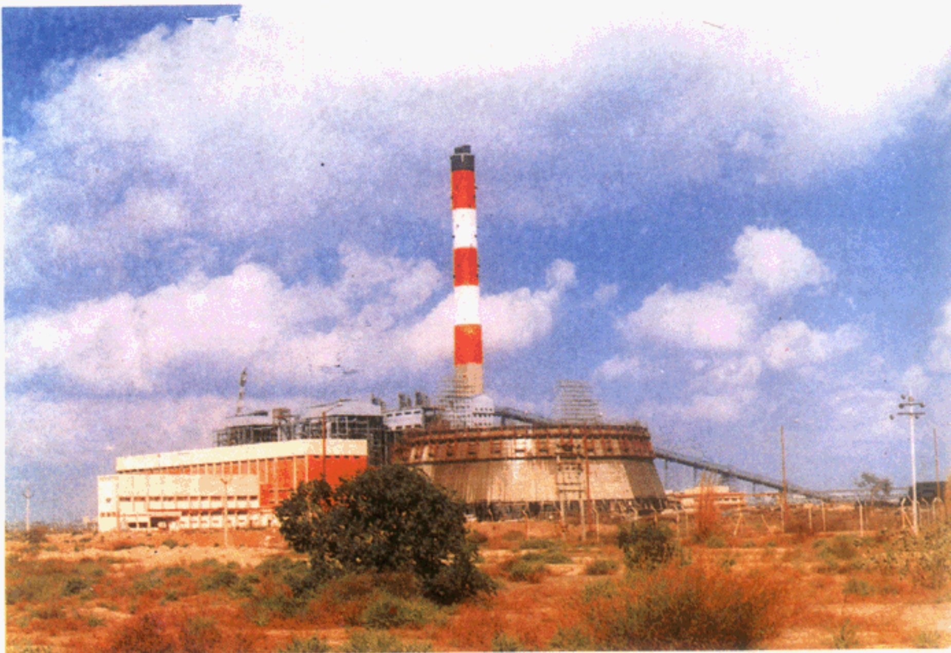
220 M High Chimney for PSEB at Lehra Mohabbat, Distt. Bhatinda
