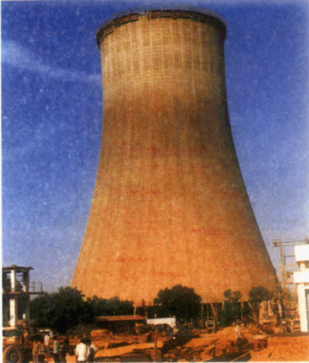
Cooling Tower at Gandhi Nagar for Gujarat Electrical Board
