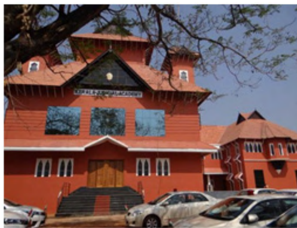
Mechanical block, NIT Jote (Arunachal Pradesh)
