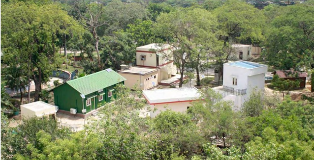
Panoramic view of the Housing Technologies Demonstration Park established at Hindustan Prefab Limited, New Delhi.
