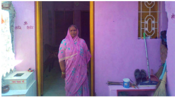
Completed house under BLC component of PMAY(U) in Gumla, Jharkhand
