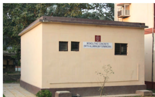
Monolithic Concrete Construction System using Aluminum formwork
