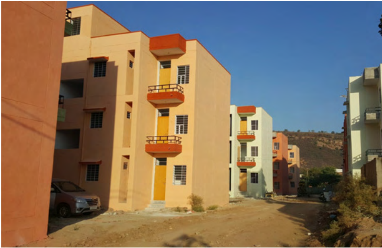
AHP Houses under RAY at Chittorgarh, Rajasthan
