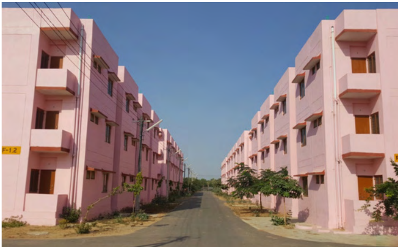
Completed IHSDP Houses at Bheelwara, Rajasthan
