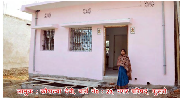
Geo-tagging of BLC Houses, Jharkhand
