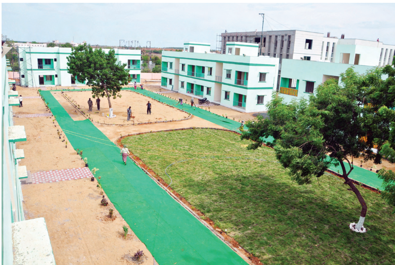
Demonstration Houses constructed using Glass Fibre Reinforced Gypsum (GFRG) Panel Technology by BMTPC at Saraswathi Nagar, Venkatachalam Mandal, SPS Nellore District, Andhra Pradesh
