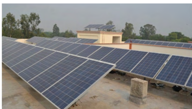
Roop top solar panels at Hindustan Prefab Limited Office cum Factory Complex at Jangpura, New Delhi
