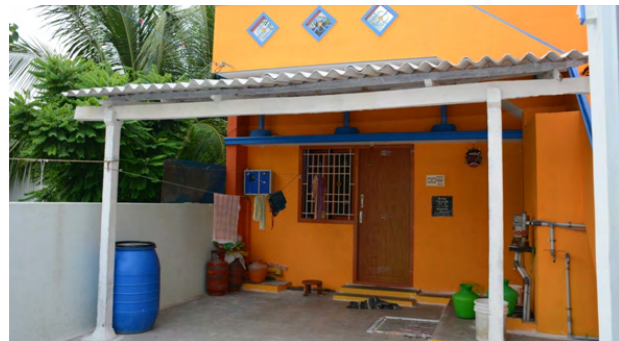
Completed House under BLC-PMAY(U), Tamil Nadu
