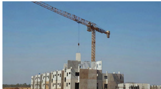
PMAY(U) Houses built with Pre-fabricated material at Naya-Raipur, Chhattisgarh
