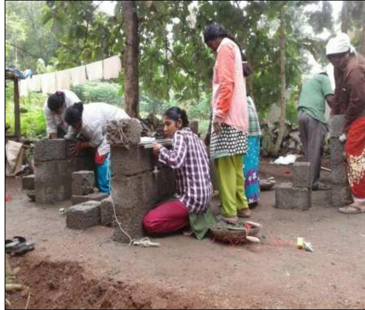
Practical – Construction using cement bricks
