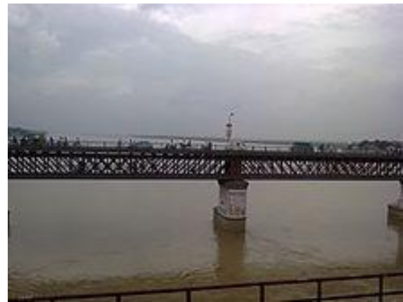
Picture 2- 3 : View of River Ganges from Kanpur Railway bridge
