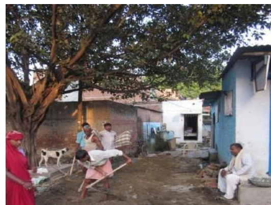
Picture 3- 10 : Construction workers
