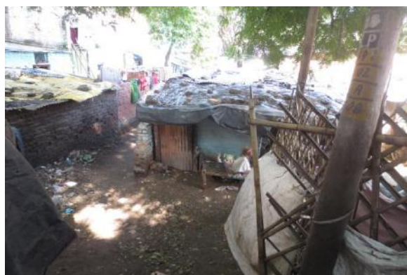
Picture 3- 8 : Katcha type housing structures in Satya Prakash slum
