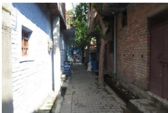
Picture 3- 21 : Non-Motorable Pucca internal road to a slum, Kanpur
