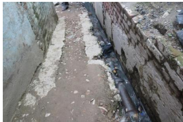
Picture 3- 16 : View of broken drainage pipeline in a slum, Kanpur
