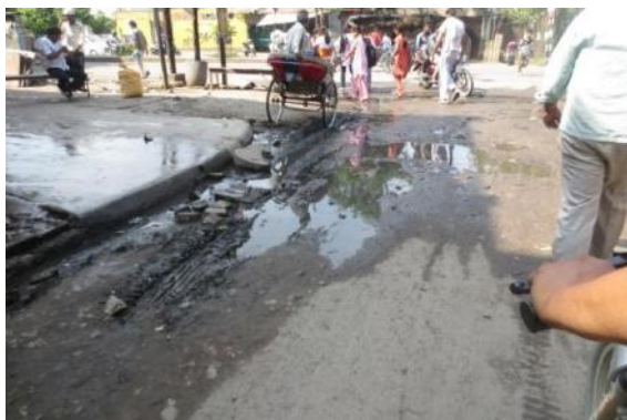
Picture 3- 19 : Motorable Katcha approach road to a slum, Kanpur
