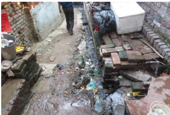
Picture 3- 15 : View of Choked storm water drain in a slum, Kanpur
