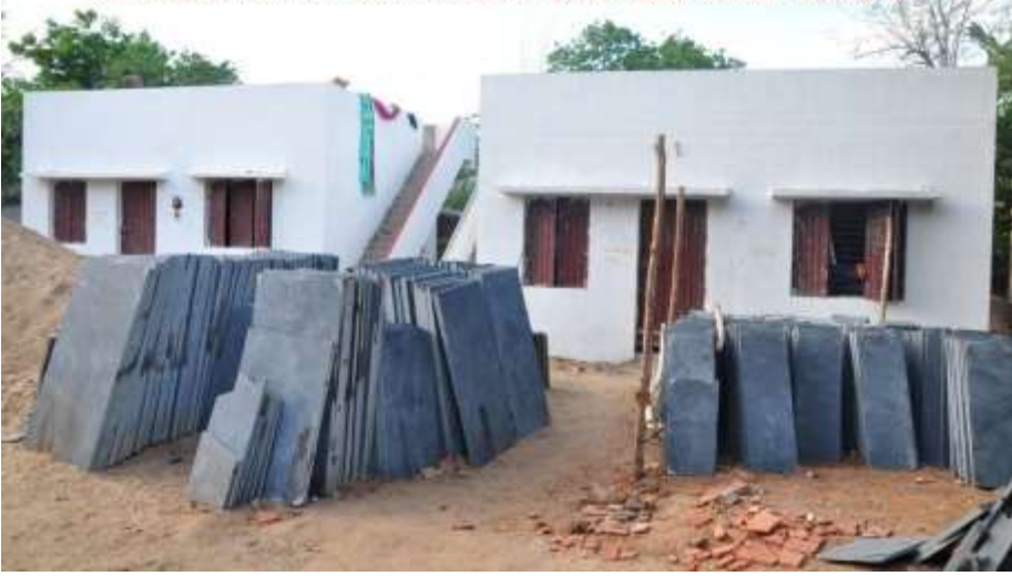
TAMILNADU SLUM CLEARANCE BOARD CONSTRUCTION OF 305 HOUSES AT KARIKALAN STREET UNDER RAY
