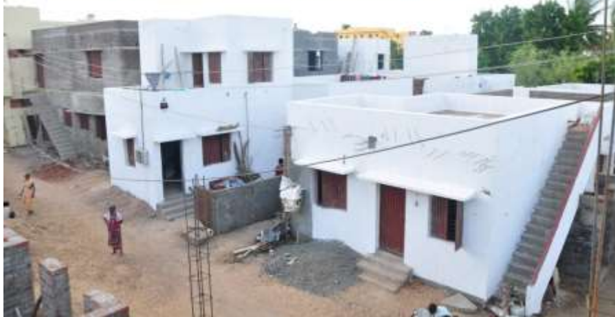
TAMILNADU SLUM CLEARANCE BOARD THIRUCHIRAPPALLI DIVISION 01.09.2014 CONSTRUCTION OF 305 HOUSES AT KARIKALAN STREET UNDER RAY
