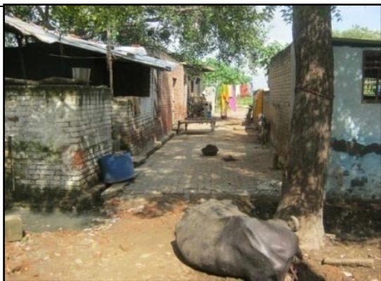
Picture 3-5 : Kolhai slum Demolished house
