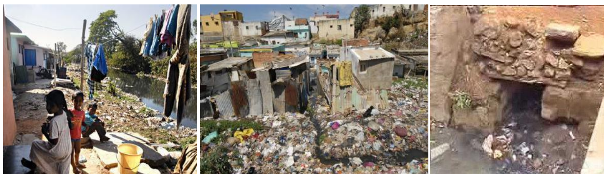
Picture 3-11 : Clearance of Drains in slums
