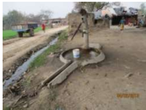
Picture 3-16 : Hand Pump in Rota-w.no-57
