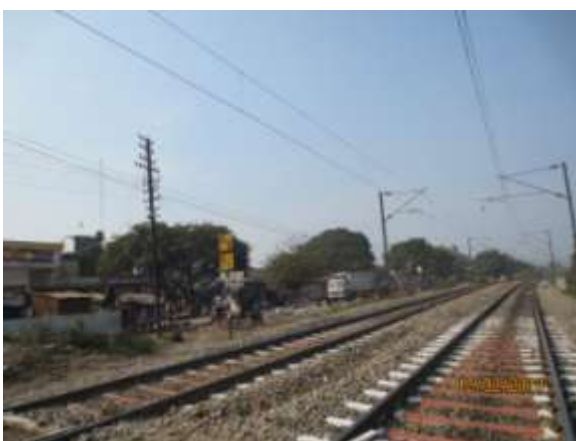
Picture 3-3 : Railway track in the vicinity of Bakargunj-w.no-24 Slum
