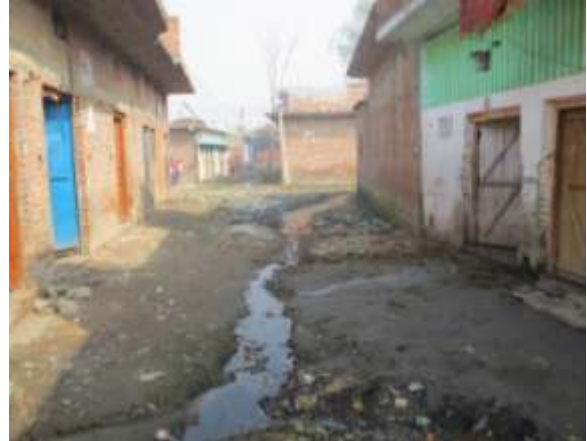
Picture 3-30 : Non-Motorable katcha internal road in Nadhosi-w.no-17
