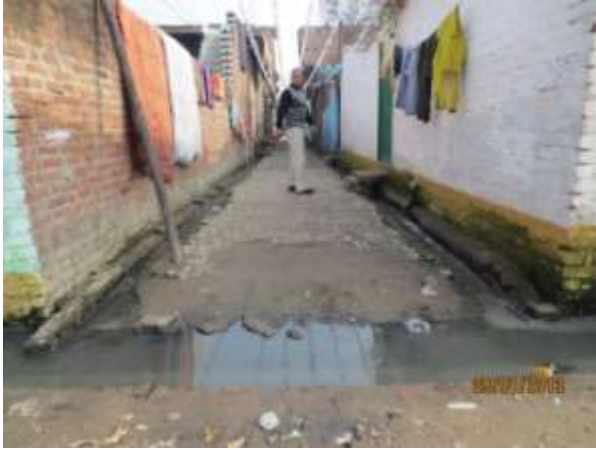
Picture 3-17 : open drainage in Reahpura choudary-w.no-49
