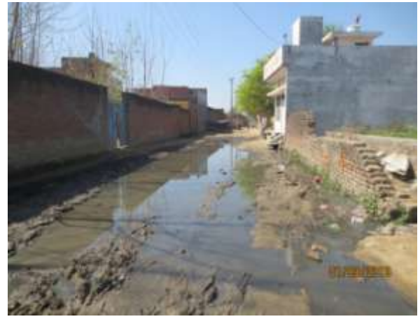
Picture 3-20 : Open drainage in thulasher pur-w.no-7
