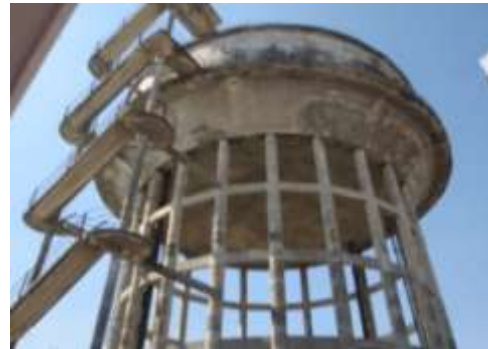
Picture 3-14 : Over headed reservoir in Ezaz nagar-w.no-67
