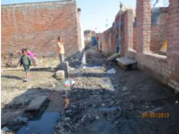
Picture 3-29 : Non-Motorable katcha internal road in Maheshpur-w.no-57
