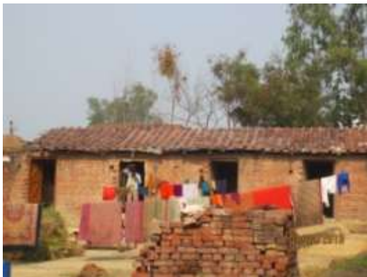
Picture 3-9 : Semi-Pucca Housing in Mathurapur-w.no-34
