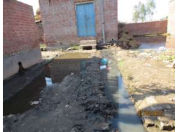
Picture 3-18 : Open drainage in Atariya-w.no-57
