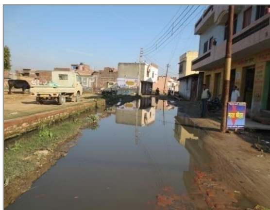
Picture 3-1 : Stagnant of rain water in Janakpuri slum
