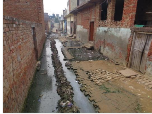
Picture 3-14 : Overflow of storm water in Indira colony
