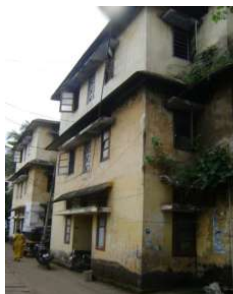
Figure 0-2: Dilapidated apartment in the colony
