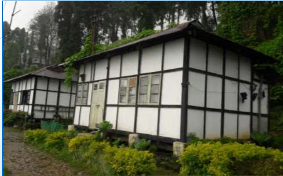
1 BHK, Constructed by Nagaland PWD (W&H) for 4 th Grade Staff
