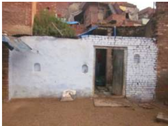
Picture 3-10: Katcha housing structures in Barahi taula slum
