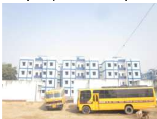
Picture 3-38: Private Senior Secondary school in People ka adda slum
