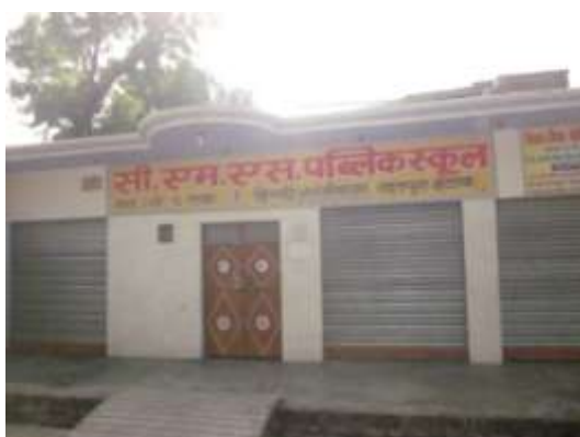
Picture 3-37: Private primary school in Rahatpura
