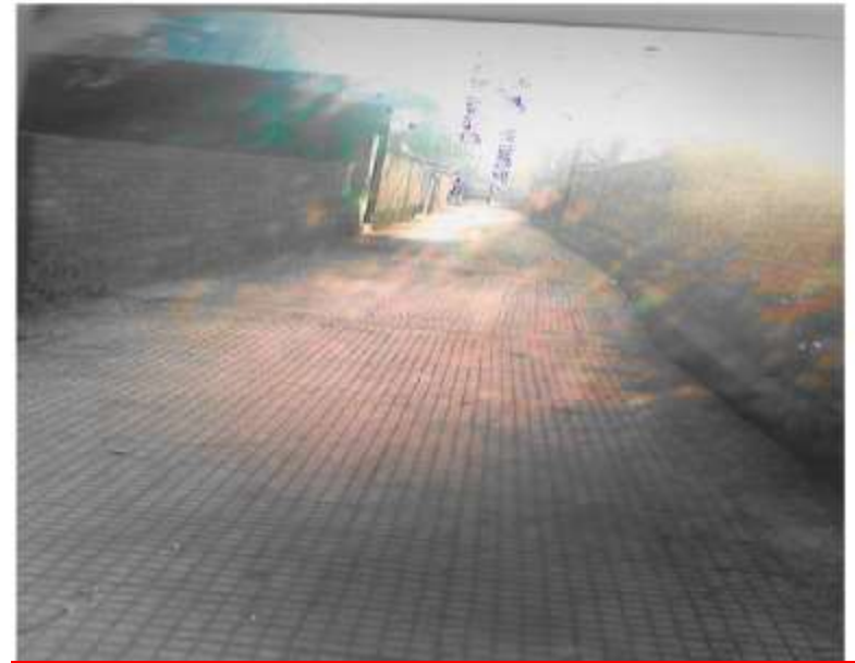
CONSTT OF TILED LANE AT MC SOPORE
