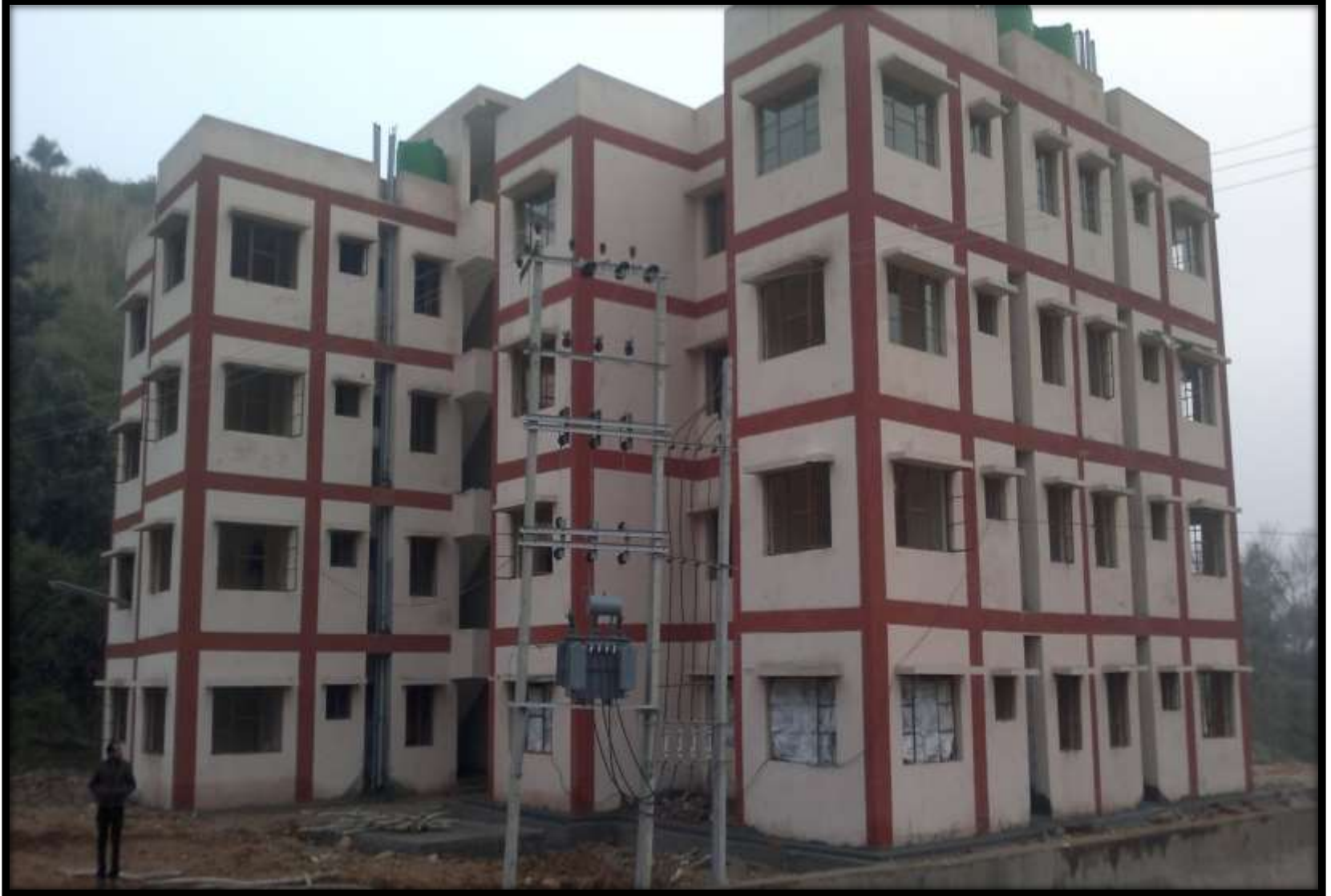
Sunjwan blocks...With electric supply
