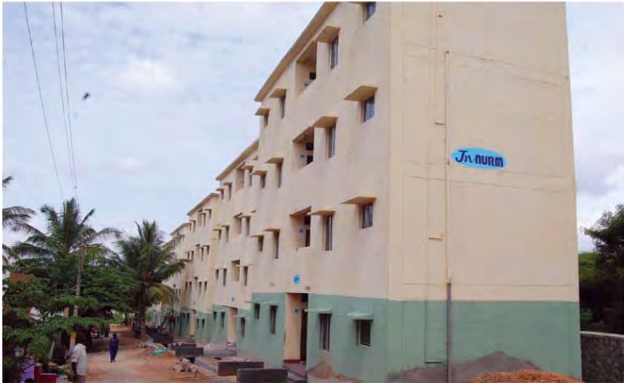
Construction of houses under BSUP, JNNURM at Mysore, Karnataka
