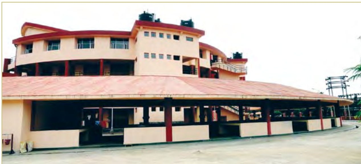
Construction of market complex for rehabilitation of vendors at Deragaon, Assam under 10% LS Scheme for North Eastern States
