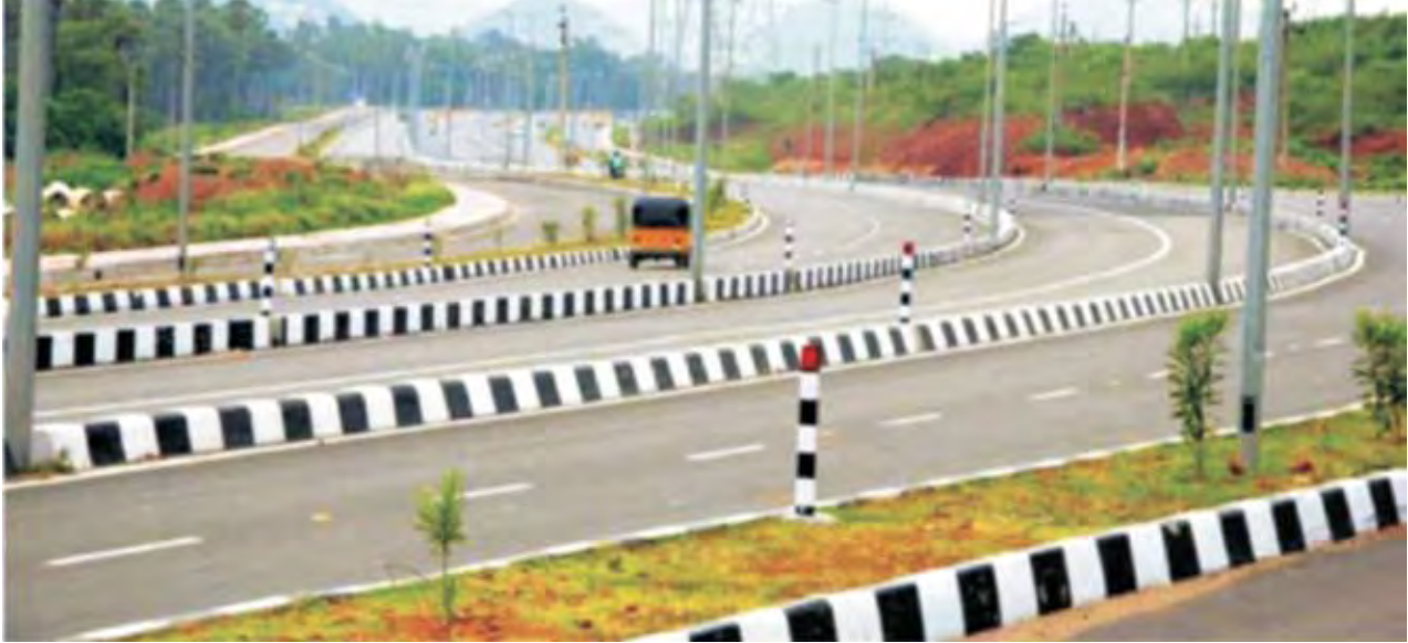
Infrastructure project funded through JNNURM, GOI BRTS-Corridor, Visakhapatnam Municipal Corporation
