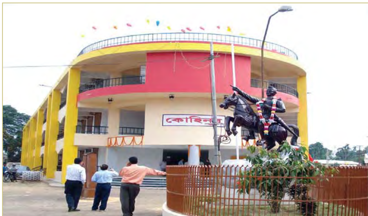
Shopping Complex for rehabilitation of evicted hawkers at Khowai Nagar panchayat, Agartala under 10% LS Scheme for North Eastern States
