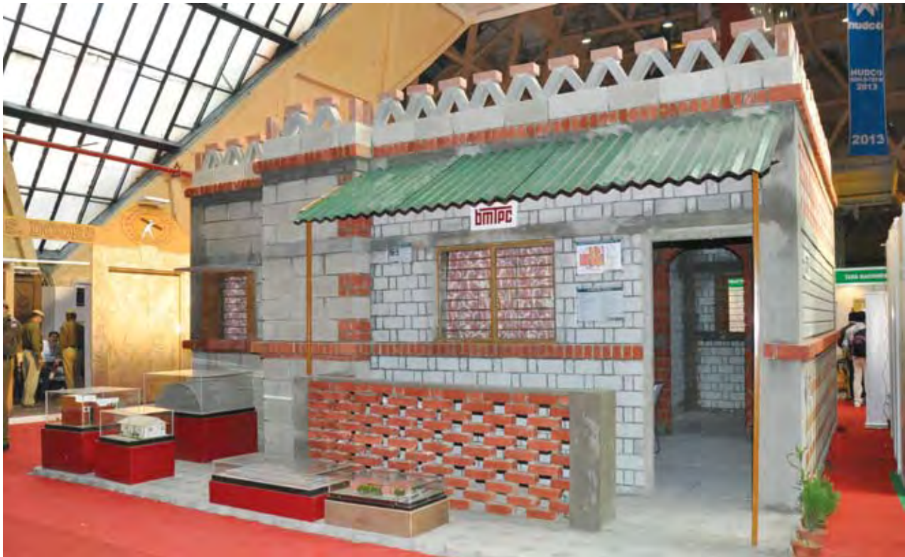
Demonstration House constructed by BMTPC to demonstrate various alternate housing technologies during the India International Trade Fair at Pragati Maidan, New Delhi from 14-27 November, 2013
