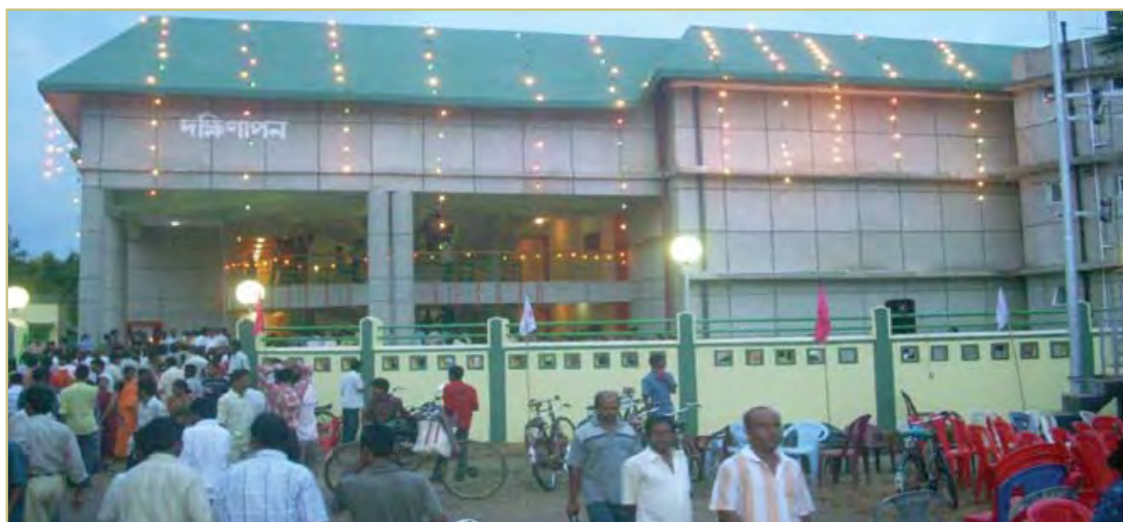
Construction of Shopping Complex for rehabilitation of evicted hawkers at Belonia Nagar panchayat, Agartala under 10% LS Scheme for North Eastern States
