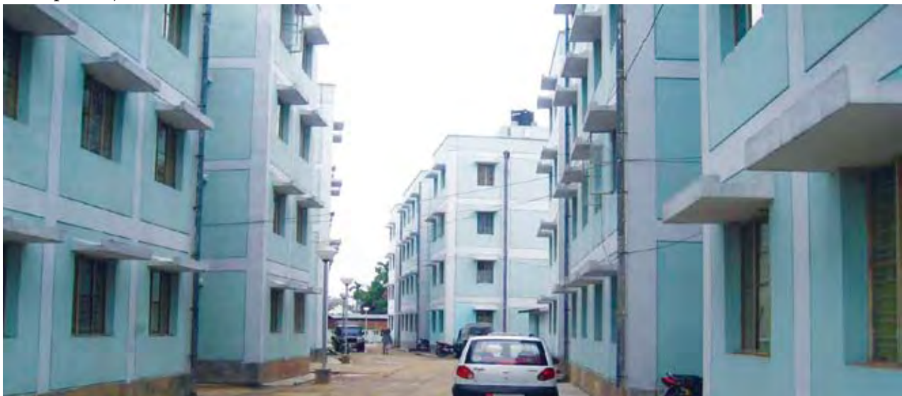
Construction of 4 storied RCC building for LIG category at Borsojai, Guwahati under 10% LS Scheme for North Eastern States
