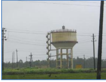
Picture 1- 31: Overhead tank, Alarwada (Ashrayya colony)
