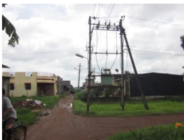
Picture 1- 60 Transformer at Ganesh nagara, Vadagaon
