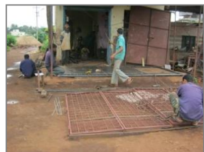
Picture 1- 26: Welding works in Rohidas nagar 4 th railway gate
