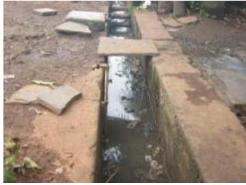
Picture 1- 41:Open drain in Rohidas nagar,4th railway gate
