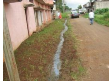
Picture 1- 43:Drain at maruthi nagar(bijapur road)
