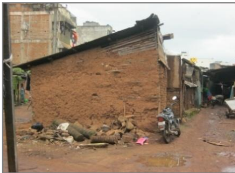
Picture 1- 6: Katcha house at Kasai galli
