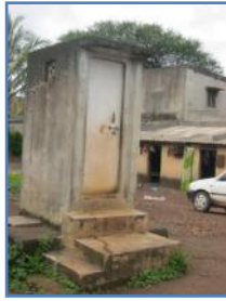
Picture 1- 44: Individual toilet in Bramhadev nagar
