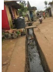
Picture 1- 40: Open drain- ramnagar waddarwadi
