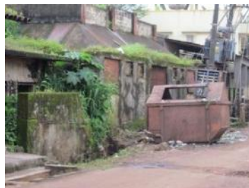
Picture 1- 54: Bin at Devang nagar, Vadagaon
