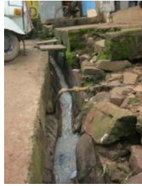
Picture 1- 42:Drainage facility in Kasai galli
