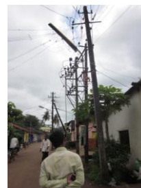
Picture 1- 61 Condition of street lights, Devang nagar, Vadagaon
