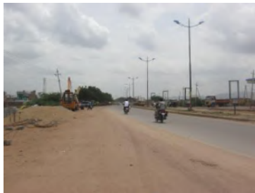
Picture 1- 15: Along the Major Transport alignment, Bandimot area
