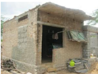
Picture 1- 26: Pucca House Under Costruction, Kaakarlahota
