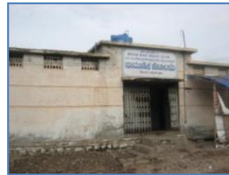
Picture 1- 44: Community toilets in Budubudu keru (Bandimot area)
