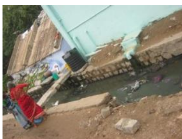
Picture 1- 38: Storm water drain in Millerpet-I
