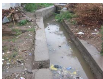
Picture 1- 39: Storm water drain at Andral slum
