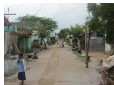
Picture 1- 40: Sewer lines passing through centre of the road, Andral Harizankeri
