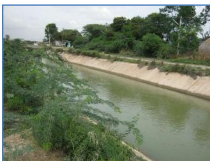
Picture 1- 21: Canal at Shanthi nagar slum
