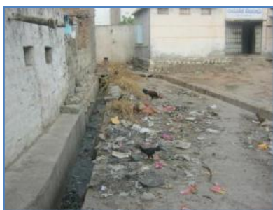
Picture 1- 41: Drainage situation in Budubudu keru Bandimot area
