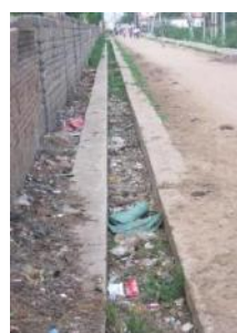
Picture 1- 42: Drainage situation in Andral slum
