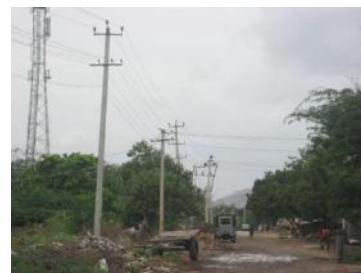
Picture 1- 50: Street lights along the road, B.Gonal
