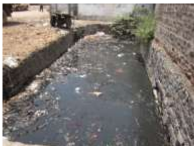
Picture 1- 8: Karl marks nagara Along major storm water Drains
