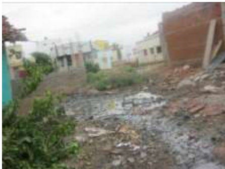
Picture 1- 12: Shivanagara slum Drainage water
