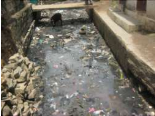
Picture 1- 37: Near vinayaka talkies slum storm water drainage
