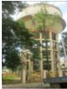
Picture 1- 31: Shekarappa nagara slum over head tank
