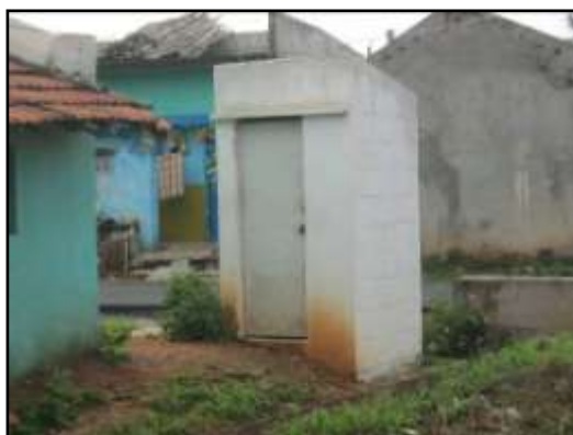
Picture 1- 41: Sriram nagar own toilets
