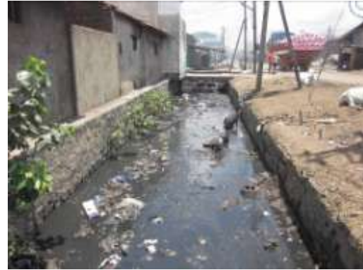
Picture 1- 38: Karlmarks nagara slum storm water drainage
