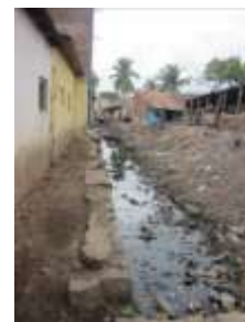
Picture 1- 9: Indiranagara, kuruchethotti Along other drain
