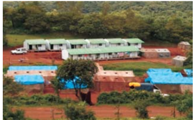
Prefab Shelters for CRPF at Belgaon (Karnataka)
