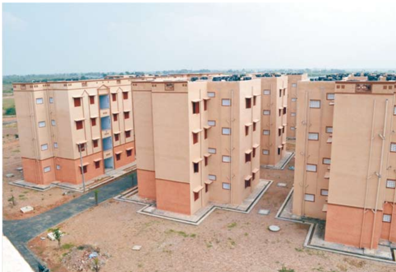
Houses built under JnNURM (BSUP) in Coimbatore, Tamilnadu
