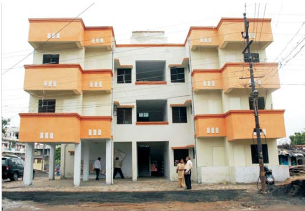
Houses built under JnNURM (BSUP) in Nagpur, Maharashtra
