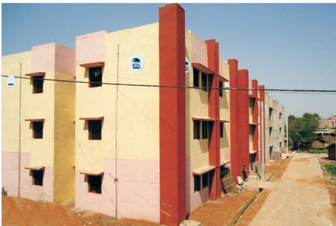
Houses built under JnNURM (IHSDP) in Bilaspur, Chattisgarh
