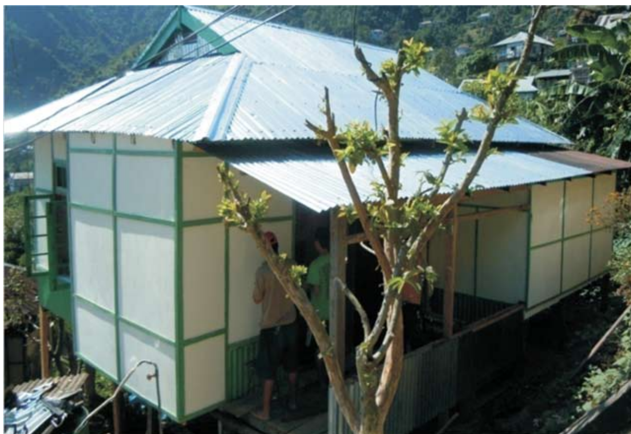
Houses built under JnNURM (IHSDP) in Mizoram
