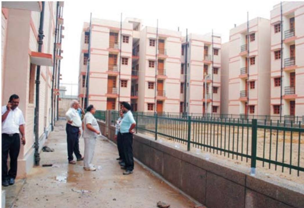
Houses built under JnNURM (BSUP) in Dwarka, Delhi
