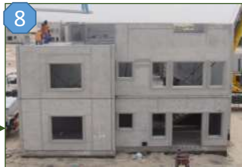
7 First Floor Wall Panel Erection
