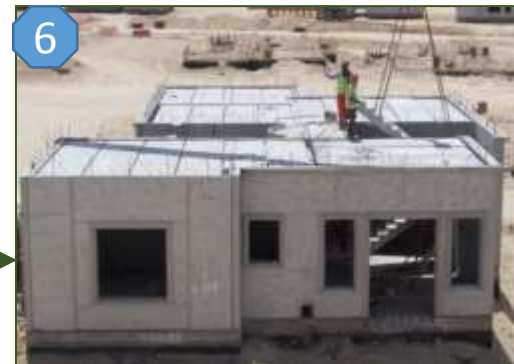
3 Ground Floor Slab Panel Erection
