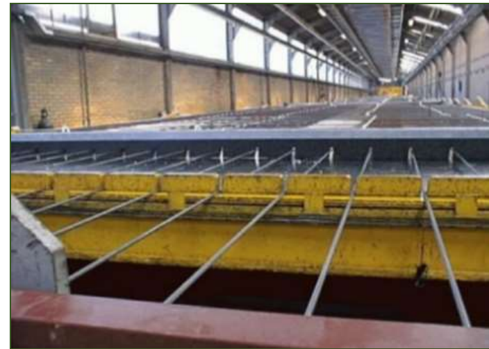
Manufacturing of Walls and Slabs
