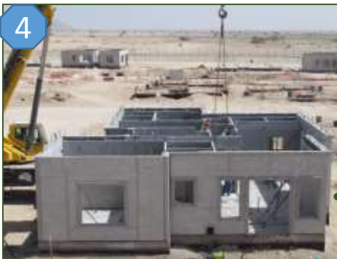
4 Ground Floor Slab Panel Erection
