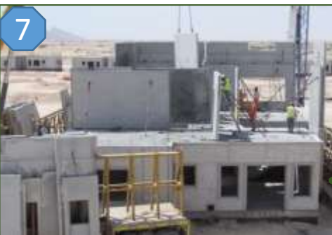
7 First Floor Wall Panel Erection
