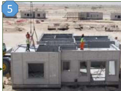
4 Ground Floor Slab Panel Erection
