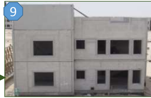
8 Two Floor Completed
