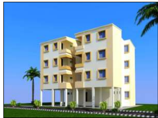
Side View of Cluster (Common sharing side walls with dead facade)
