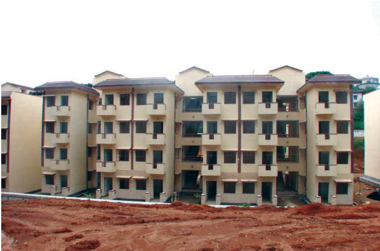
Completed Dwelling Units under JnNURM (BSUP) at Agartala, Tripura
