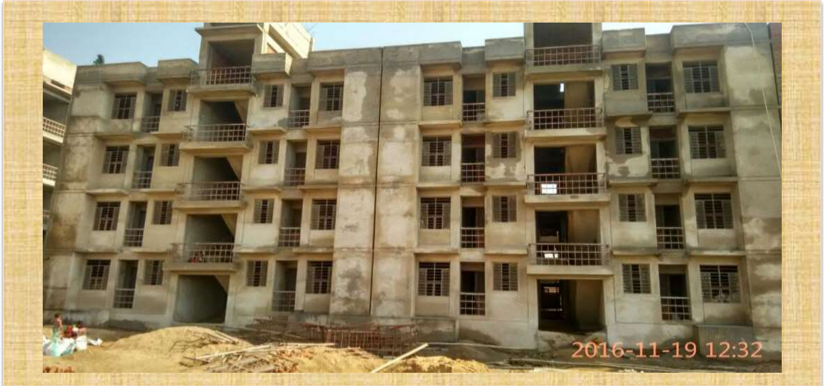
Housing Units in Budh Vihar for Relocation - Alwar
