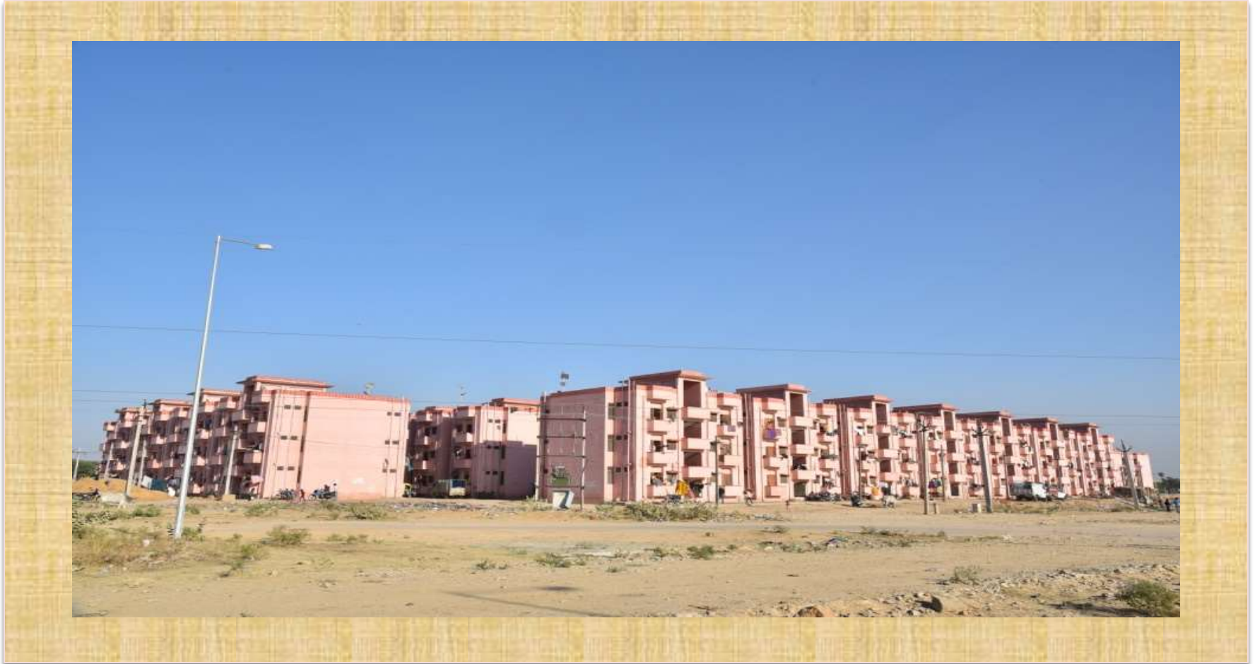
Housing Units in Kiron Ki Dhani - Jaipur
