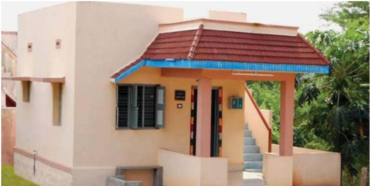
Single storied house constructed under JnNURM (IHSDP) in Pallavarayan Patti, Melur Municipality, Tamilnadu
