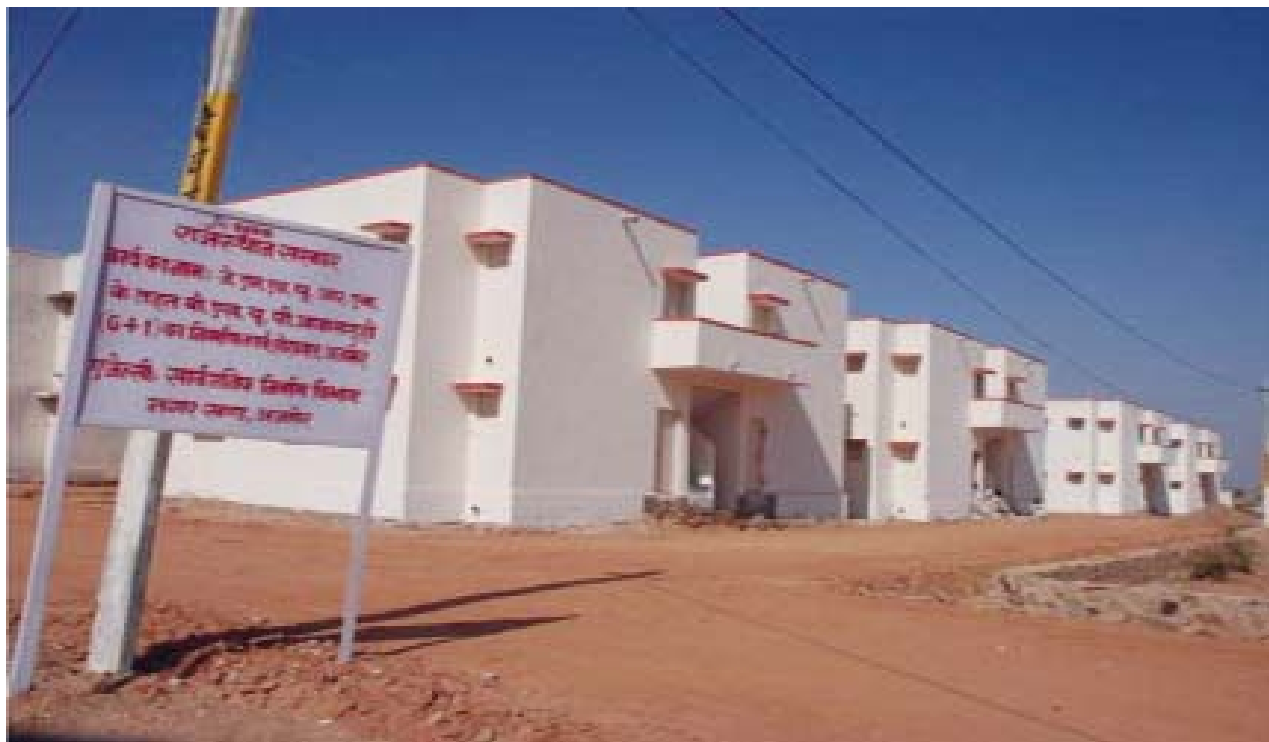
Dwelling Units nearing completion under JnNURM (BSUP) at Ajmer-Pushkar, Rajasthan
