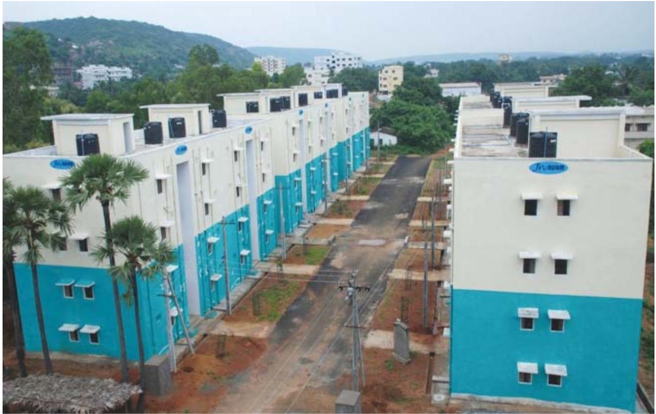
Completed Dwelling Units under JnNURM (BSUP) at Visakhapatnam, Andhra Pradesh
