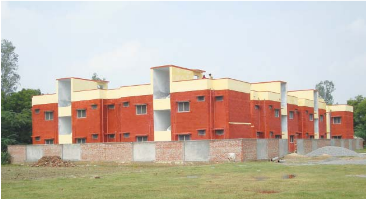
Demonstration Houses constructed by BMTPC at Amethi, Sultanpur, Uttar Pradesh
