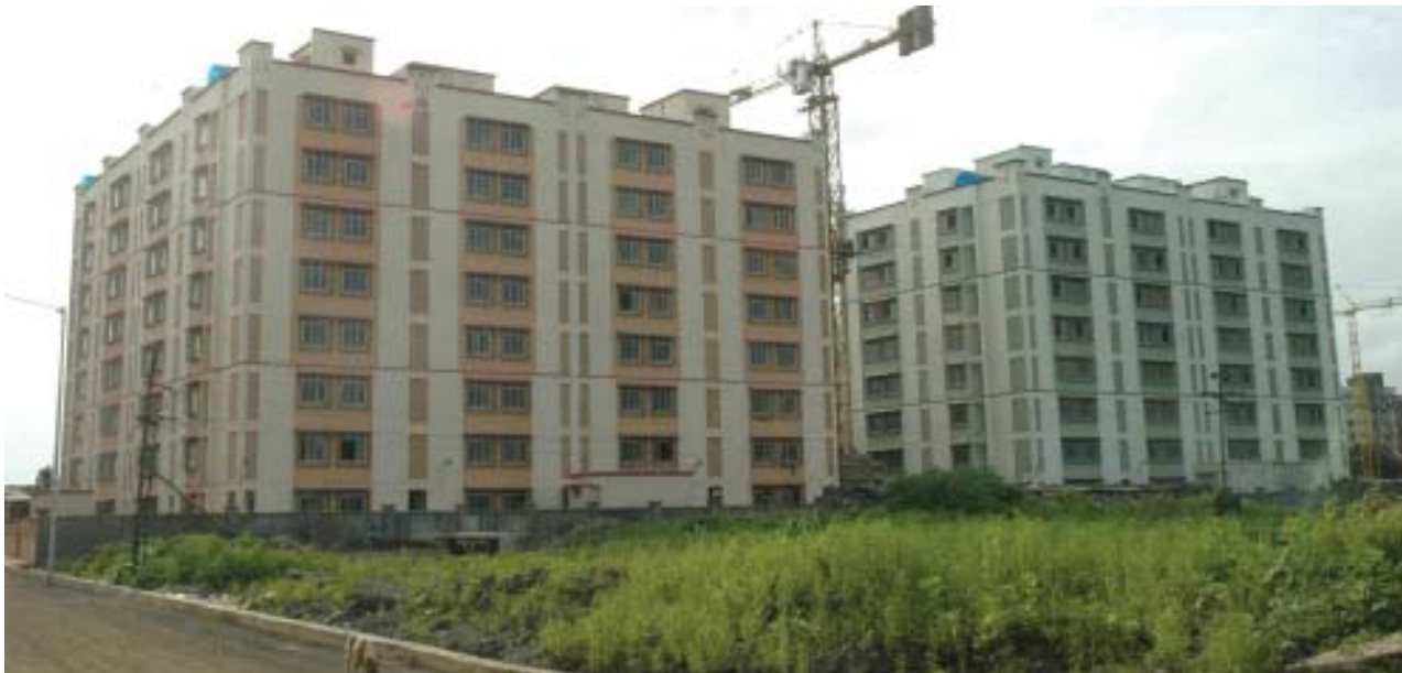
Dwelling Units constructed under JnNURM (BSUP) in Malvani (Malad), Mumbai, Maharashtra
