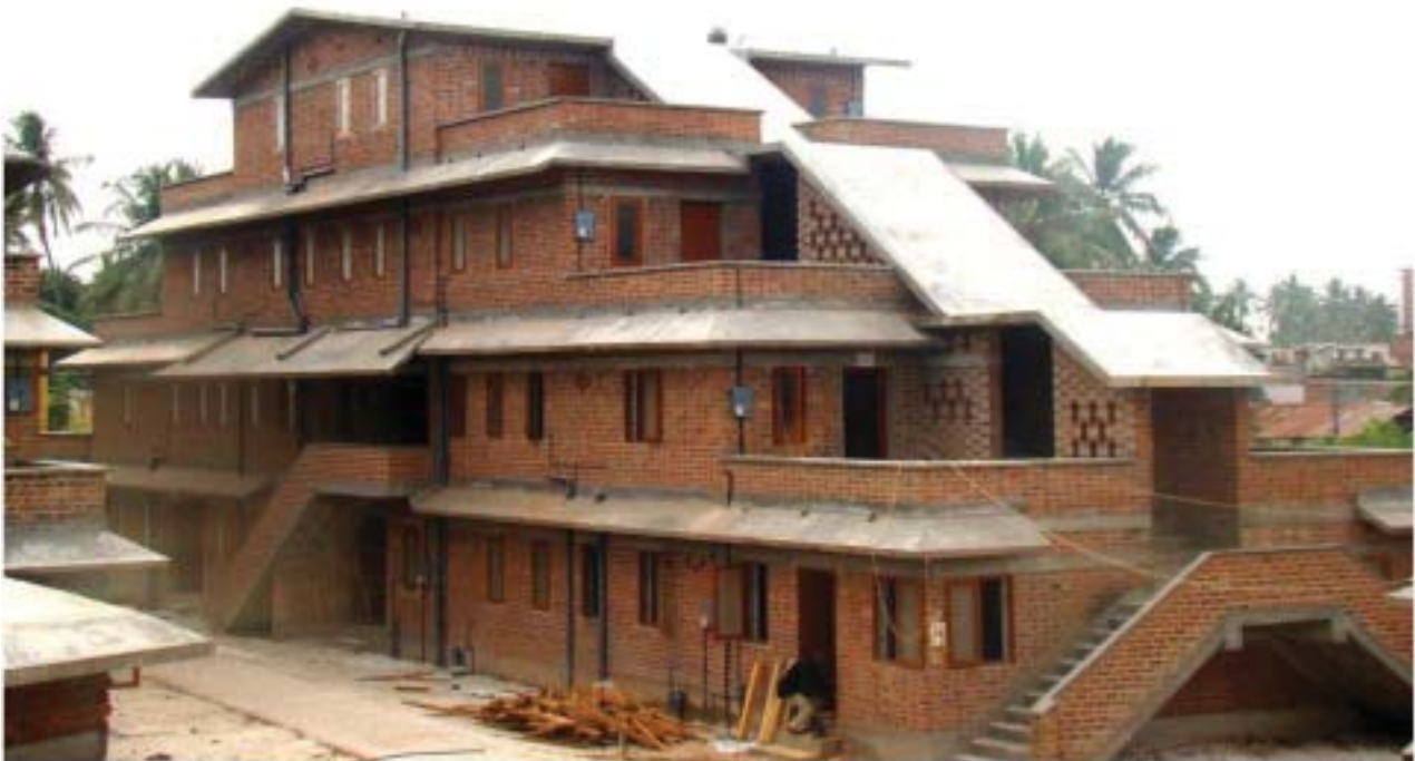
Completed and allotted housing cluster under JnNURM (IHSDP) at Karimadon Colony, Kerala
