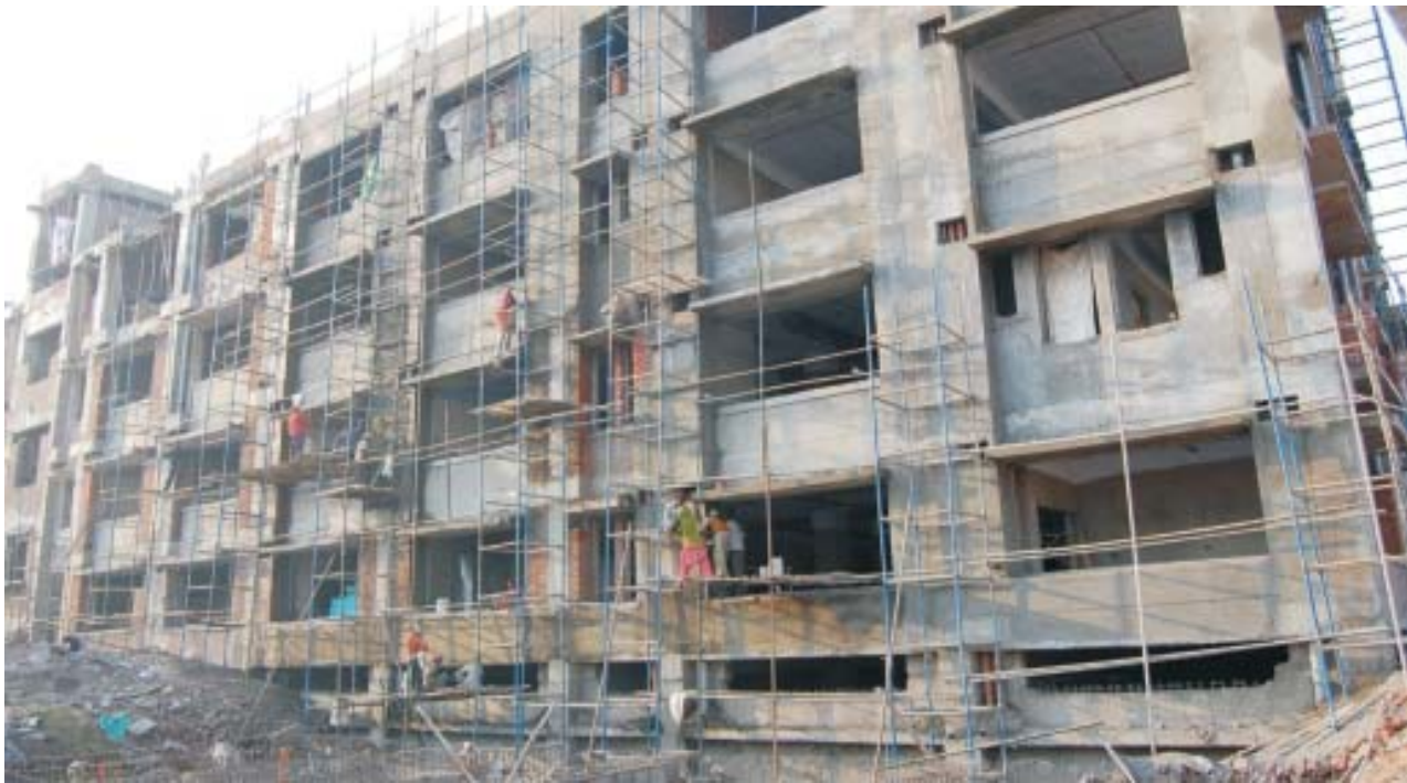
Construction of 100 Bedded Hospital at Baddi (Himachal Pradesh) by HPL
