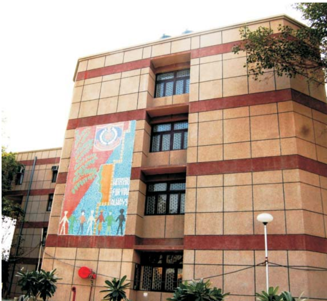
Construction of Police Station for Delhi Police, Delhi by HPL
