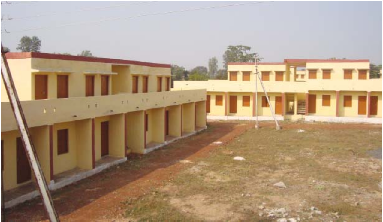
Demonstration Houses under VAMBAY constructed by BMTPC at Bilaspur, Chhatisgarh
