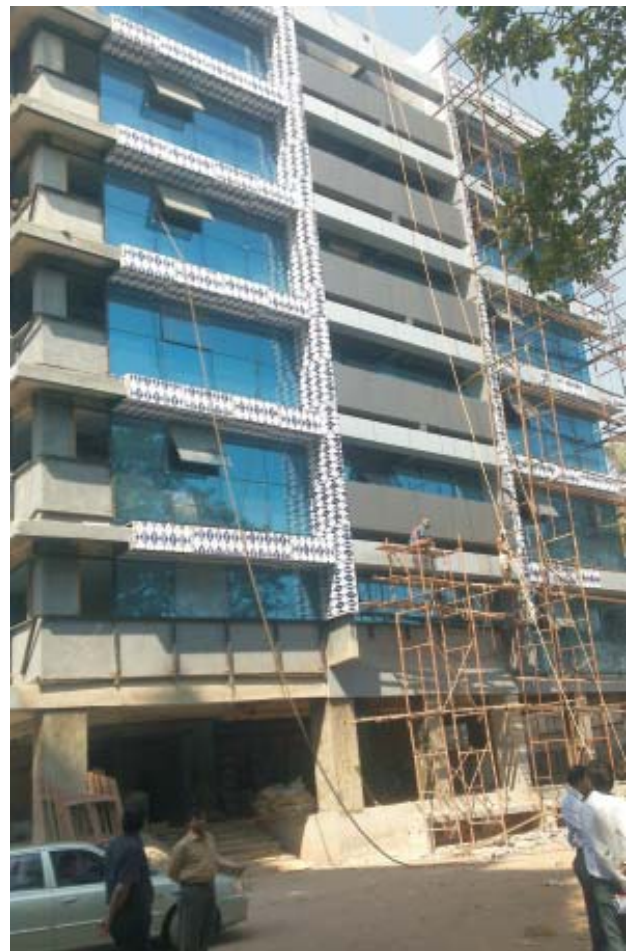
Retrofitting Work of Regional Office, ESIC Building, Lower Parel, Mumbai by HPL
