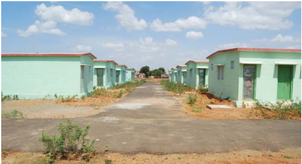
Demonstration Houses under VAMBAY constructed by BMTPC at Trichi, Tamil Nadu
