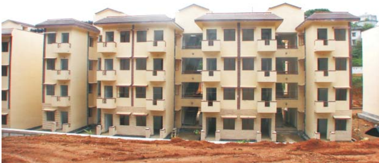
Completed Dwelling Units under JNNURM (BSUP) at Agartala, Tripura
