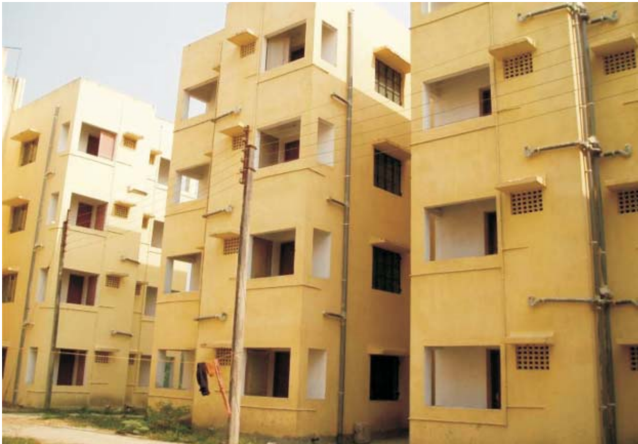
Dwelling Units under JNNURM (BSUP) at Kolkata, West Bengal
