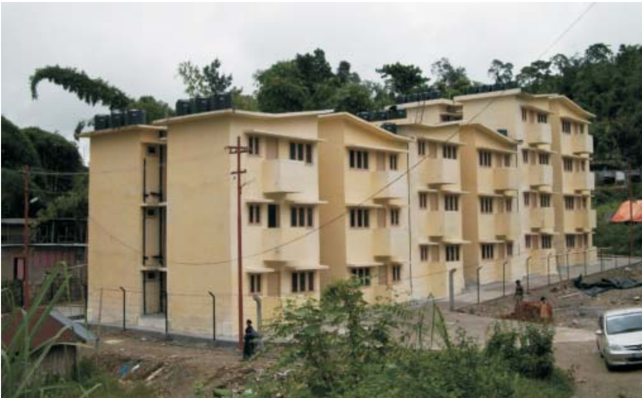
Construction of Houses for Safai Karmchari & People Below poverty line, Nirjuli, Arunachal Pradesh by HPL
