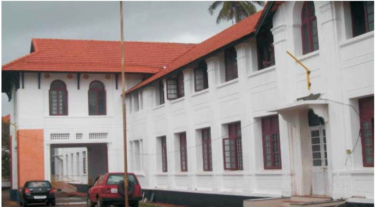
Renovation of General Hospital, Kozhikode by HPL
