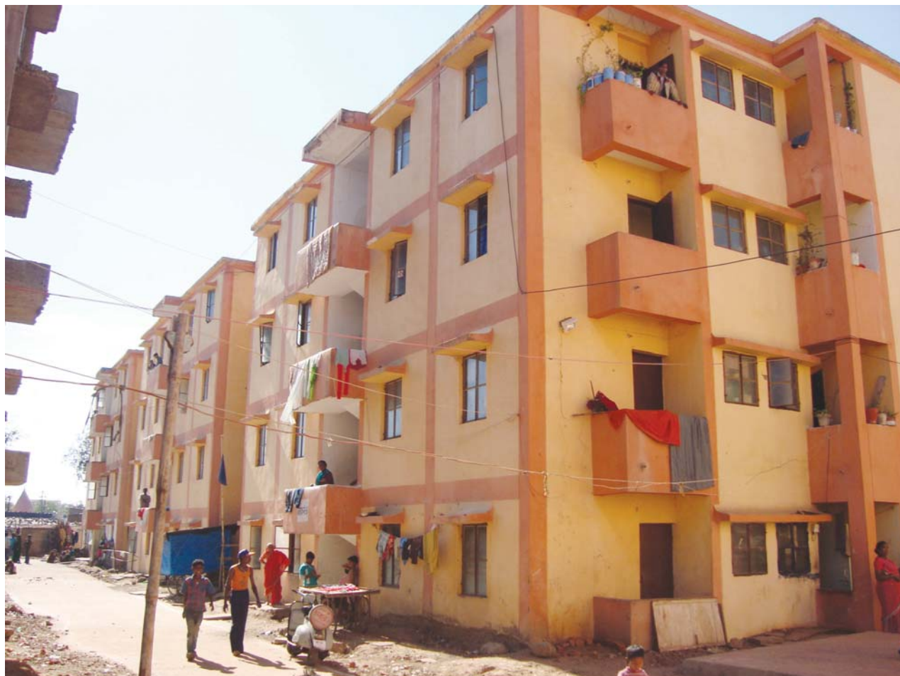
Housing under JNNURM (BSUP) in Bhopal, Madhya Pradesh
