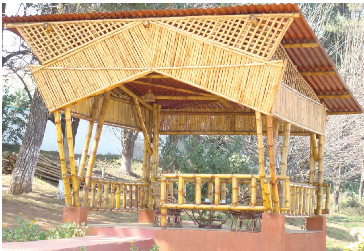
Demonstration Structure at Indian Army Holiday Home, Eastern Command Shillong, Meghalaya constructed by BMTPC using bamboo based technologies.
