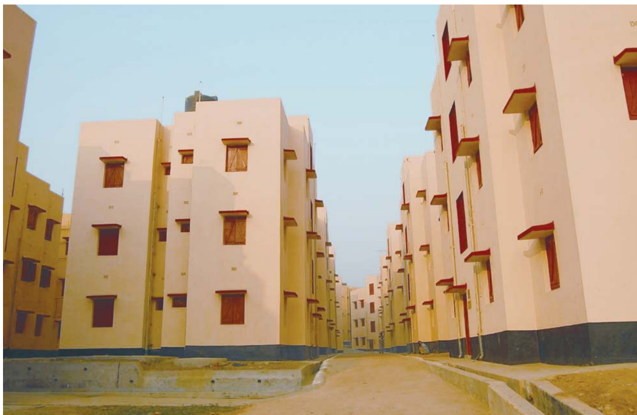
Housing Project nearing completion under JNNURM (BSUP) in Asansol, West Bengal
