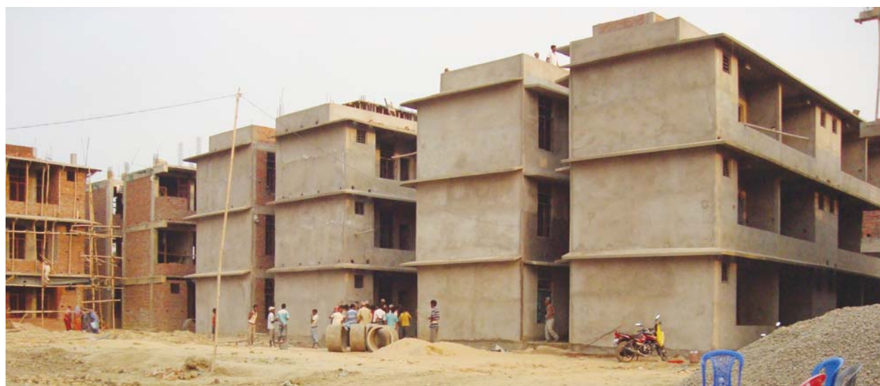
Housing Project under construction under JNNURM (IHSDP) in Dimapur, Nagaland
