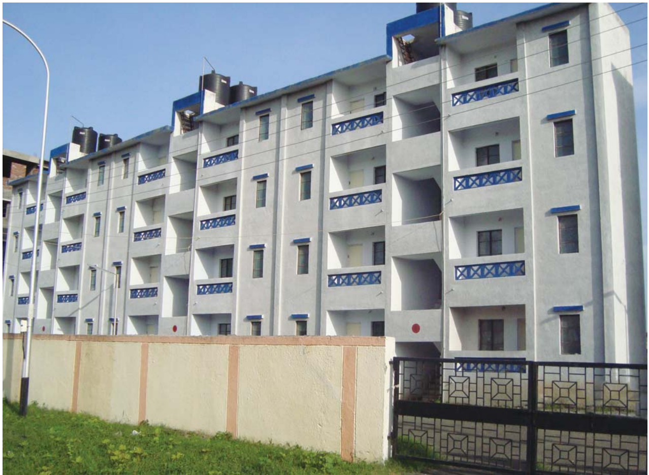
Housing Project nearing completion under JNNURM (BSUP) in Surat, Gujarat
