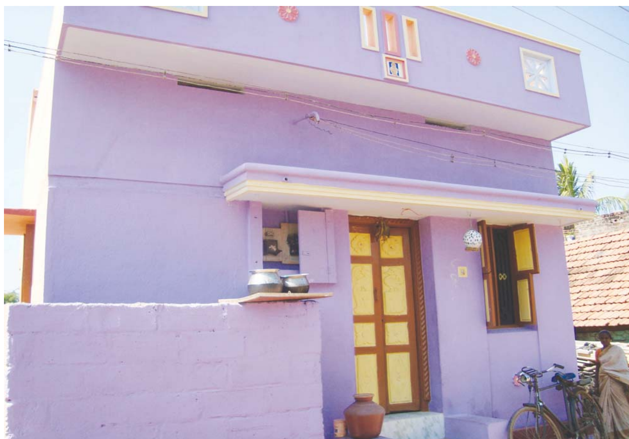
Housing under JNNURM (BSUP) in Madurai, TamilNadu
