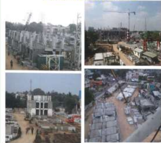
Pre-fabricated at Moorthing Street, Chennai
