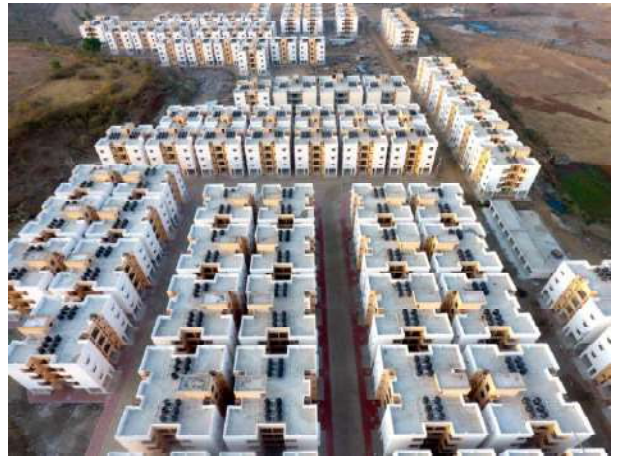
4. PMAY(U) Project in Chindwara, Madhya Pradesh
