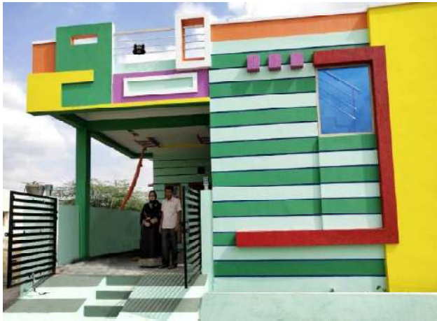
11. PMAY(U) House in Andhra Pradesh
