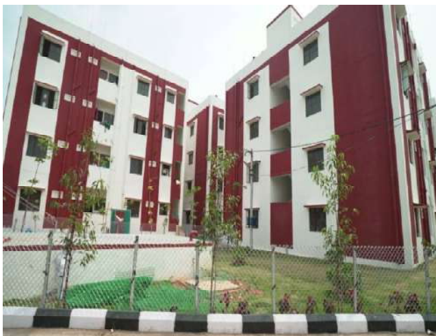
7. PMAY(U) Project in Telangana
