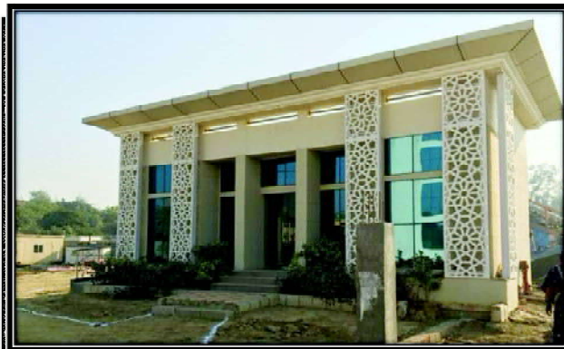
Residential-cum-Training complex for Special Protection Group at Sector-21, Dwarka, New Delhi - Rs. 466.41 crore
