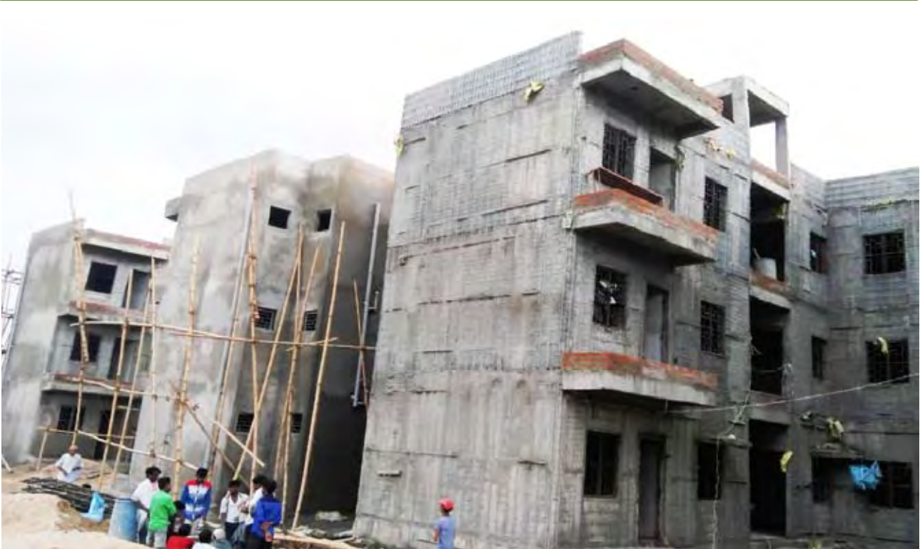
Demonstration Houses being constructed using Coffor Structural Stay in Place Formwork System by BMTPC at Bihar Shariff, Bihar
