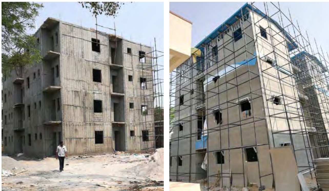
Demonstration Houses being constructed using Coffor Structural Stay in Place Formwork System (16 houses) and Light Gauge Steel Frame System (16 houses) by BMTPC at Gachibowli, Hyderabad, Telangana
