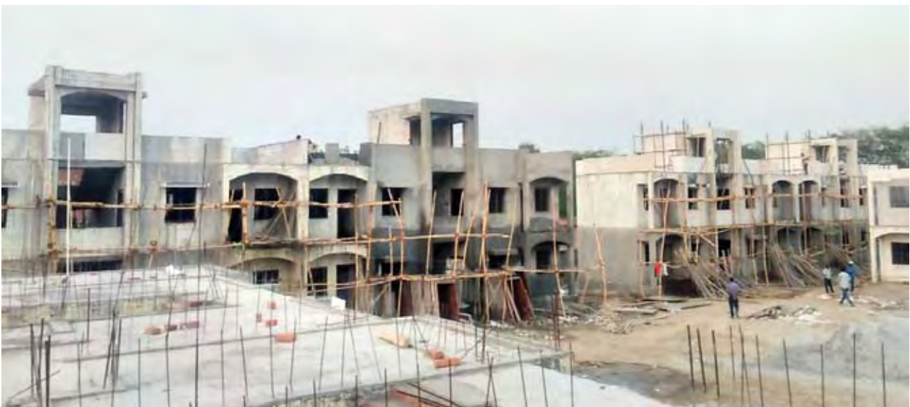
Demonstration Houses being constructed using Stay in Place EPS based double walled panel System by BMTPC at Aurangabad Jagir, Lucknow, Uttar Pradesh
