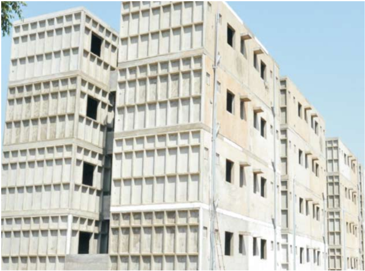
Waffle Crete System – a Technology under evaluation
