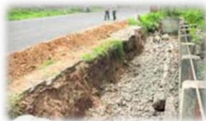
Erosion of surface lining and banks of storm water drain
