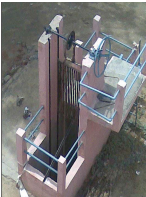
Figure 4.1 Typical Hand operated Screen Facility at Shallow Sewers in Pumping Stations
