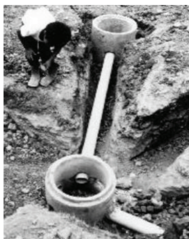
Figure 8.7 Junction chamber for simplified sewerage using larger diameter concrete pipes, used in Guatemala
