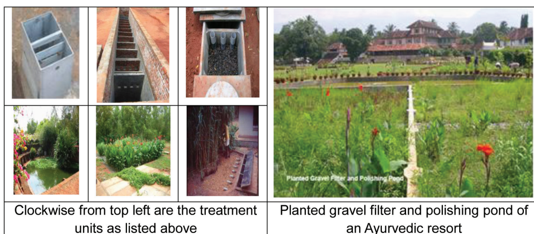
Figure 8.15 Typical DEWATS treatment plant components
