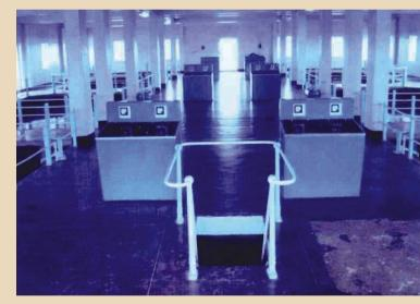
↑ Control soles for 6 nos. rapid sand filters. The 7.5 MGD water treatment plant at Mawphlang is one of its kinds in the North East to be installed with pneumatic operation.
