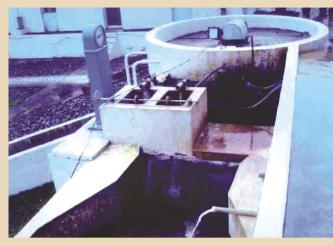
RAW WATER CHANNEL: Raw water through the 🕇 inlet channel is received in inlet chamber. The rate of flow of raw water is measured by flow meter. Alum solution from the constant dosing tank flows directly through a taper needle valve at preset dosage, which adjusts itself automatically to any change in the flow rate of water. The raw water then enters the flash mixer where the coagulant is added and rapidly mixed.
