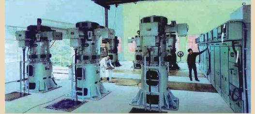
aintenance of the HT motor control centre n progress. The electric motors installed are directly fed with a voltage of 6.6 Kv.
