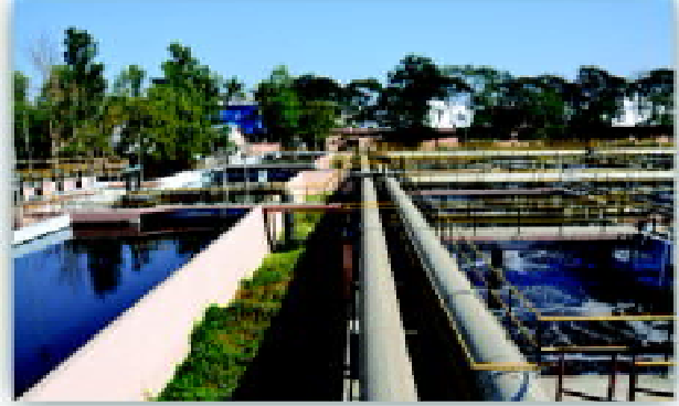
Upgradation & Augmentation of STP at Surat (Gujarat)
