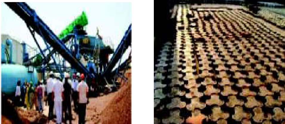
Construction & Demolition waste plant
