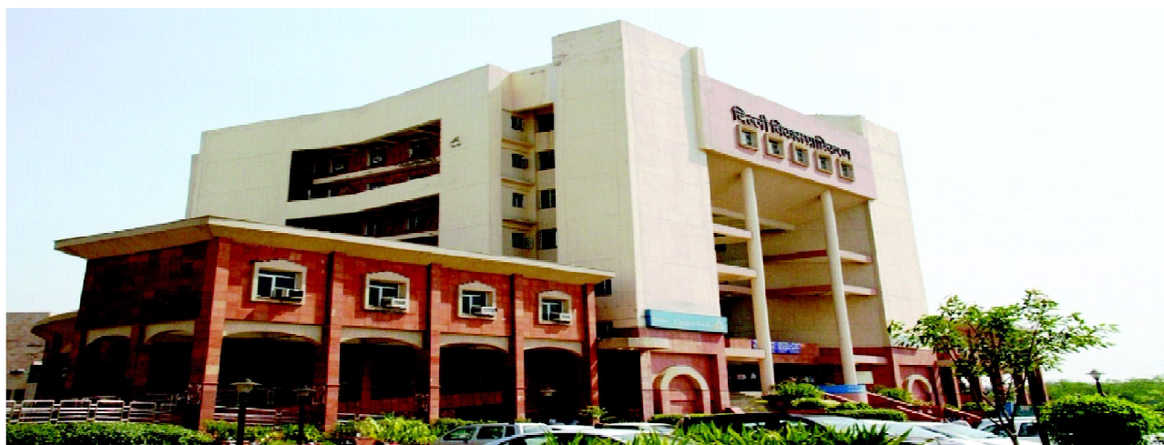
DDA Office, Madhuban Chowk
