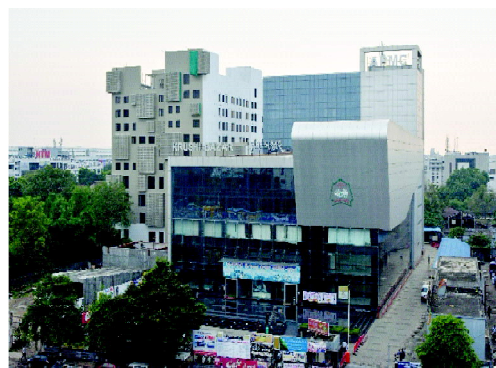
Figure 4 : APMC Building , Surat, Gujarat
