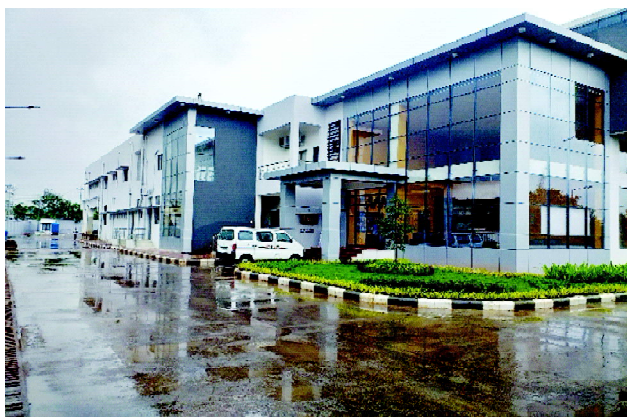
Figure 9: Kitchen Building - CSR Silvassa Project
