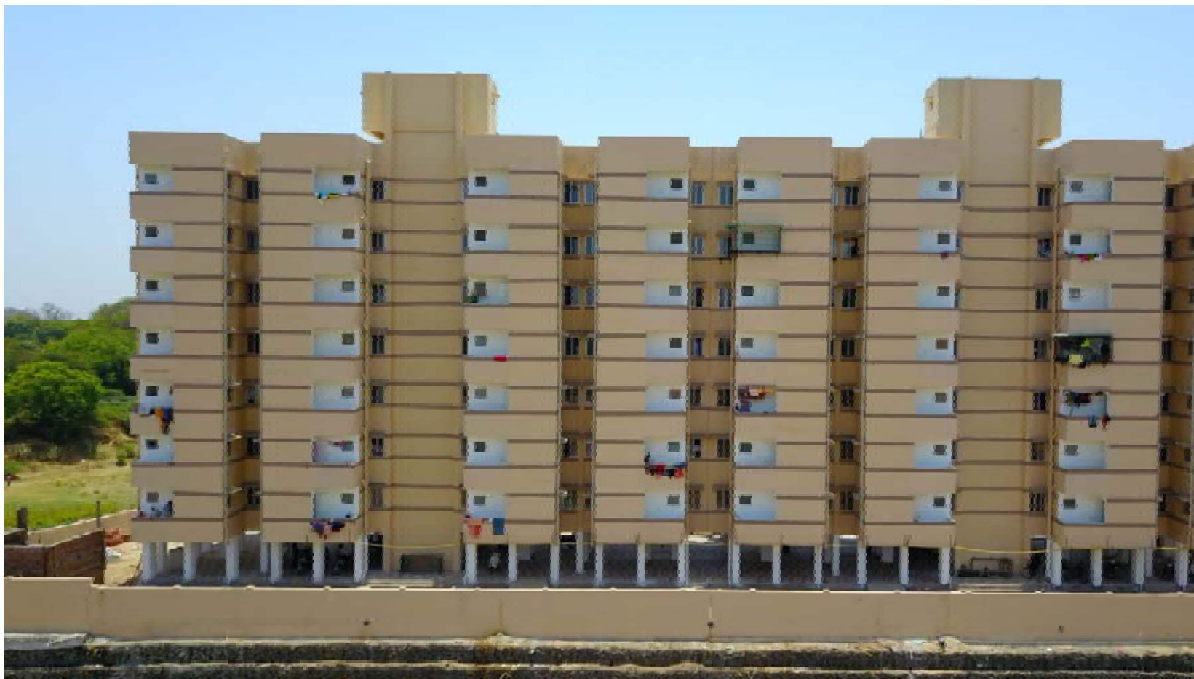
Construction of houses under ISSR in Gujarat
