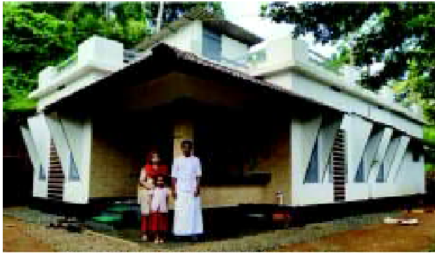
Houses constructed under BLC Project in Kerala
