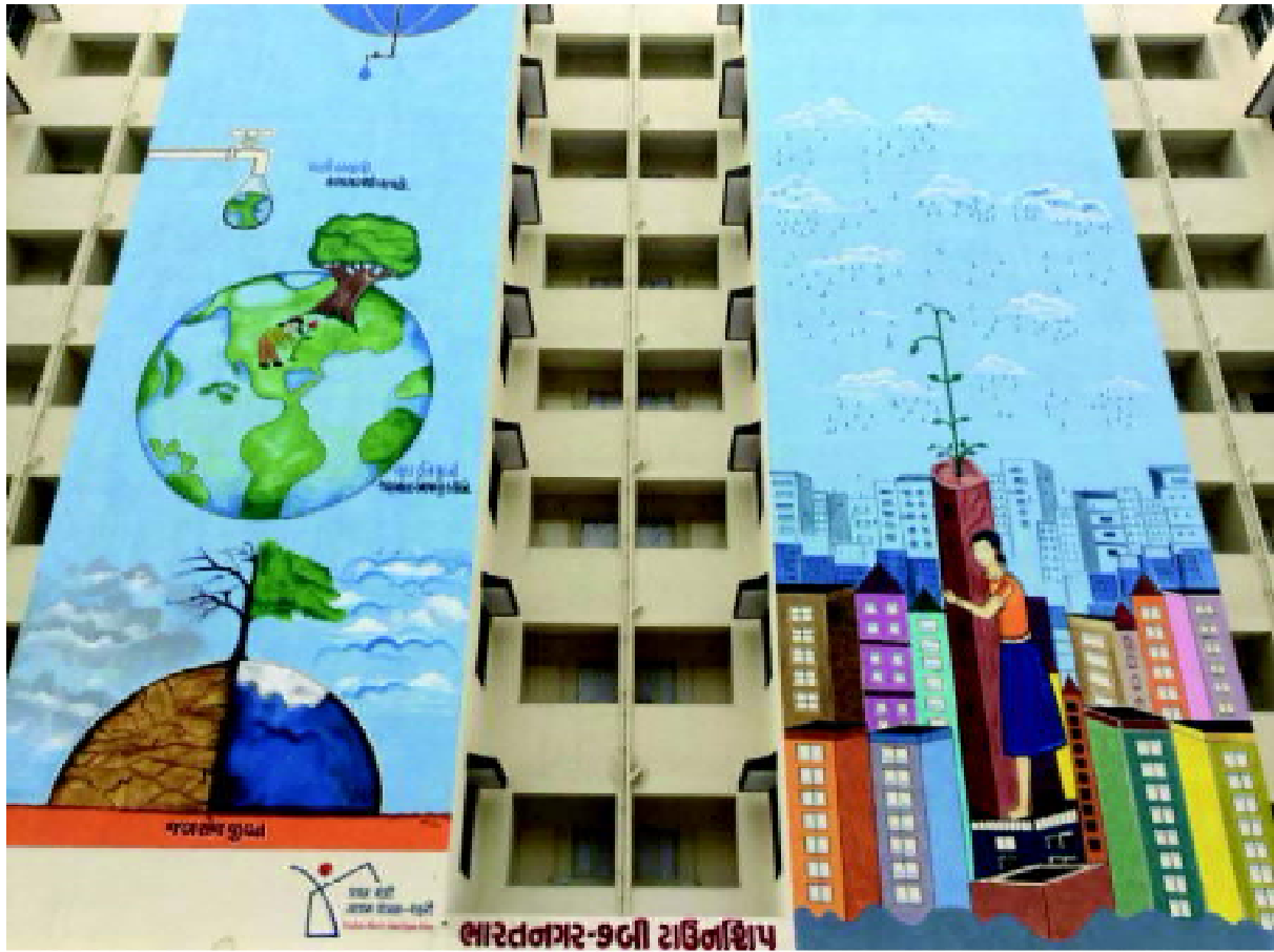
Construction of houses under ISSR in Gujarat
