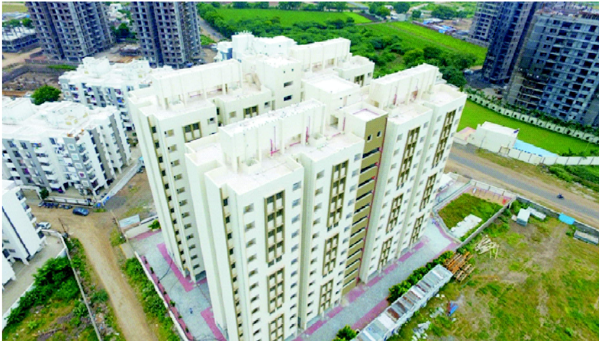
Houses constructed under AHP Project in Gujarat
