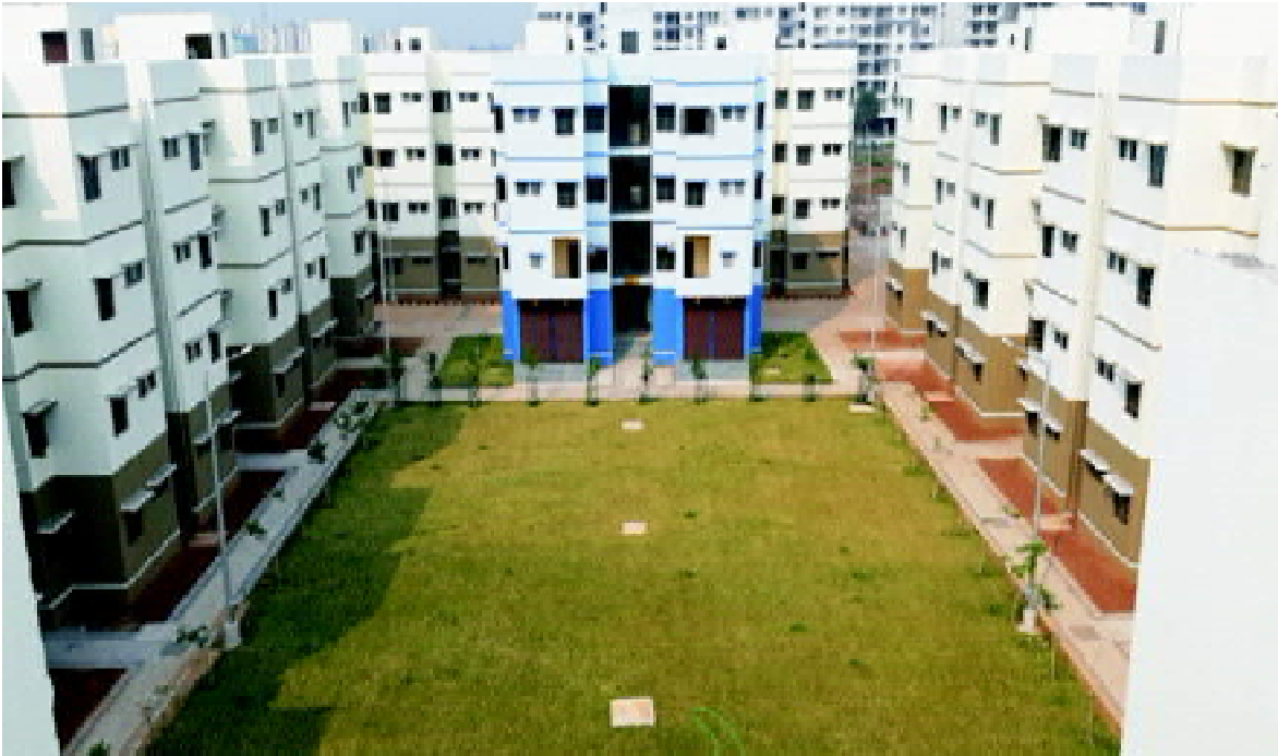
Houses constructed under AHP Project in Chattisgarh
