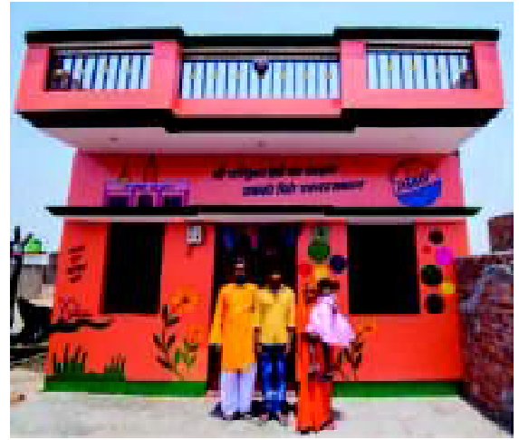
Houses constructed under BLC Project in Uttar Pradesh
