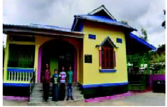
Houses constructed under BLC Project in Manipur
