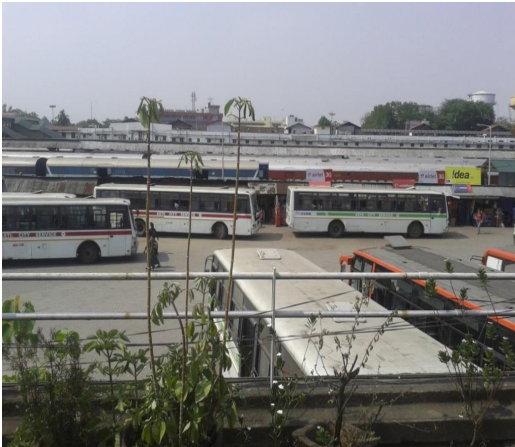
Figure 2-5: ASTC's Paltan Bazar Bus Terminal, Guwahati
