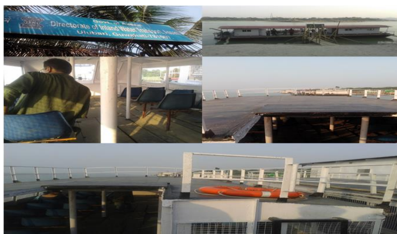
Figure 2-6: Kuchary Umananda Inland Water Transport Terminal, Guwahati
