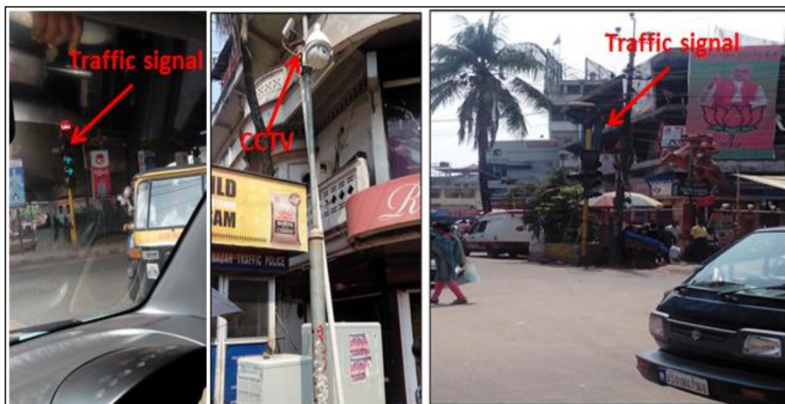
Figure 3-1: View of Traffic Signal and CCTV Cameras, Guwahati
