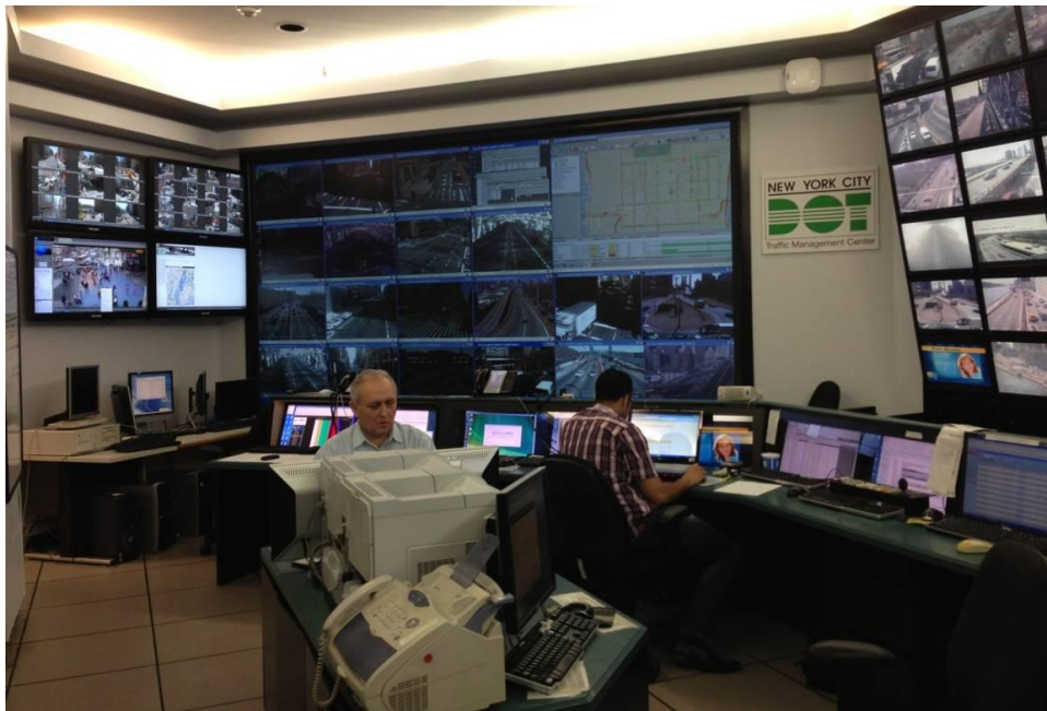
Figure 4-1: Joint Traffic Management Centre – Signal System (New York)
