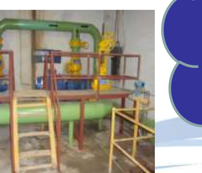
Safe working platforms
