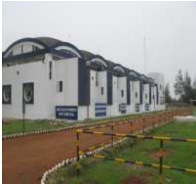
Changed over view of WTP
