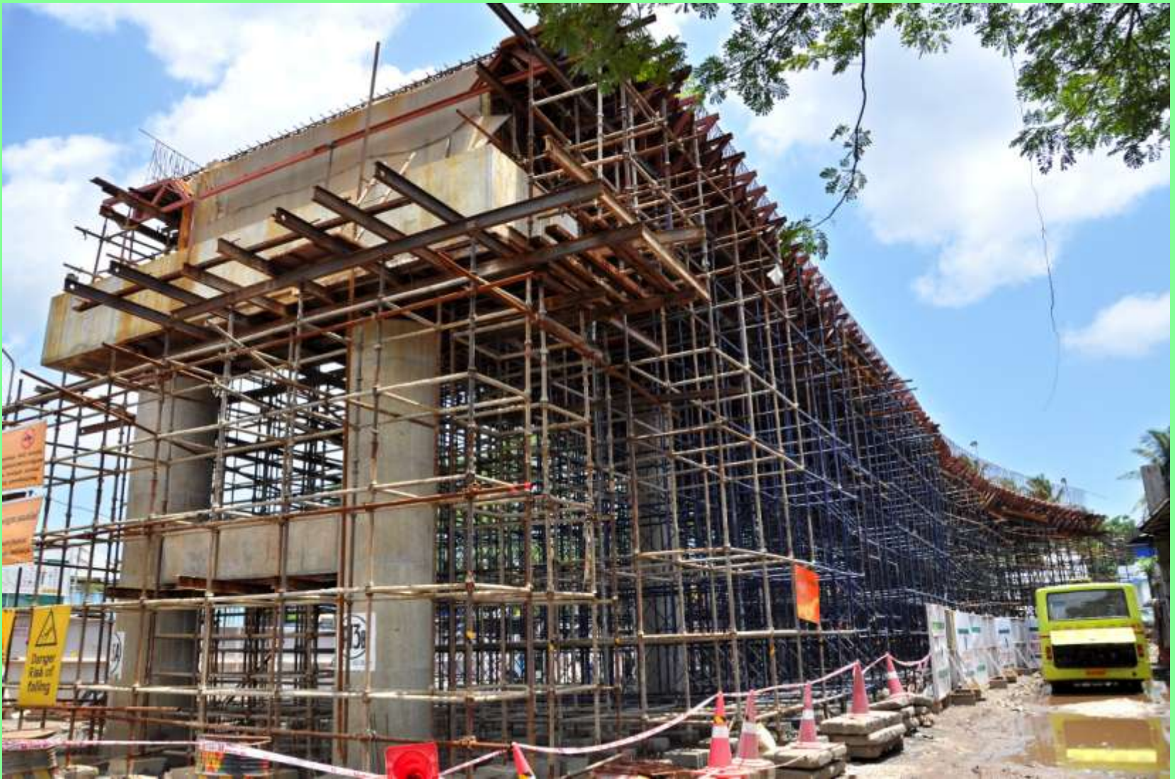
Construction of Salim Rajan ROB
