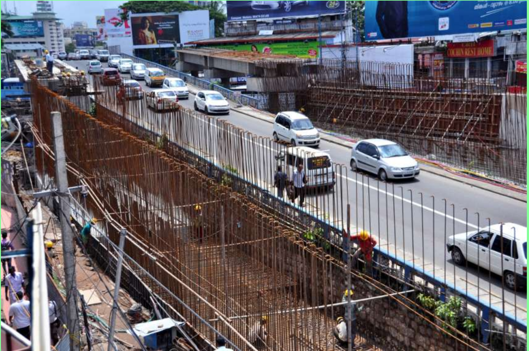
Rebuilding of North ROB
