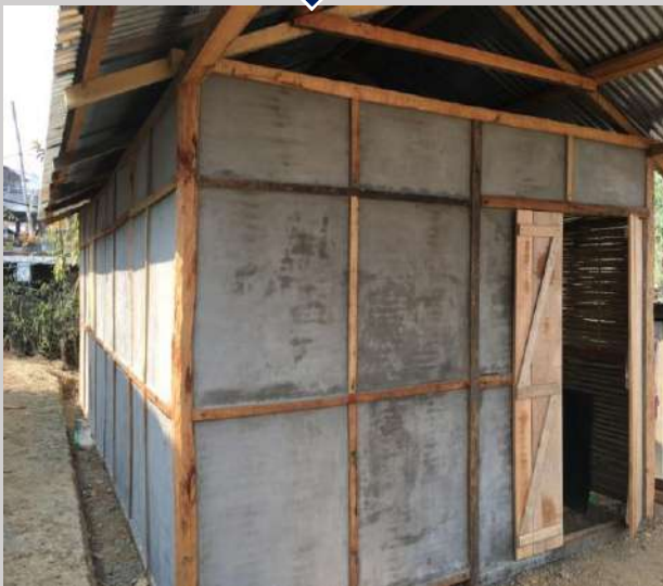
Cement Plaster on Bamboo Split
