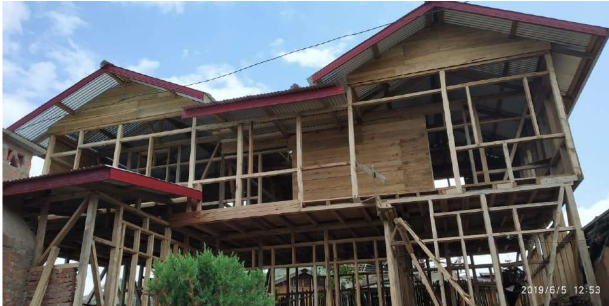
Wooden Houses constructed under BLC - New Houses, Shamator Town
