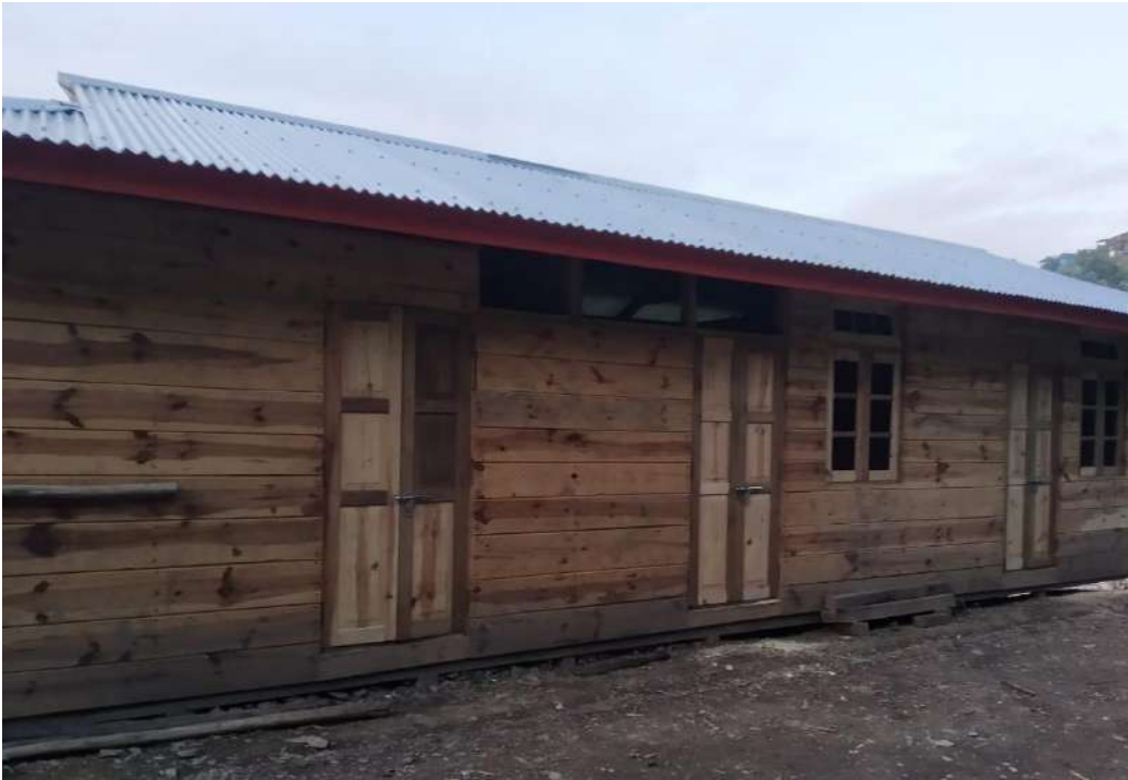
Wooden Houses constructed under BLC - New House at Kiphire Town
