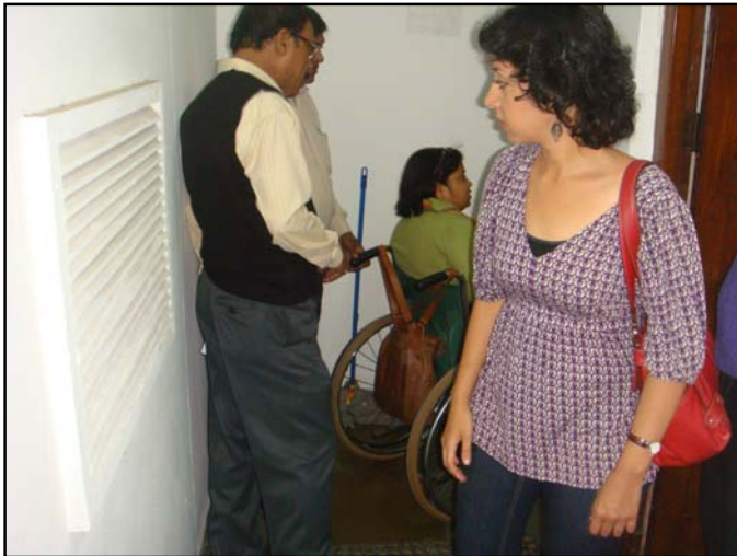
Accessible toilet under construction
