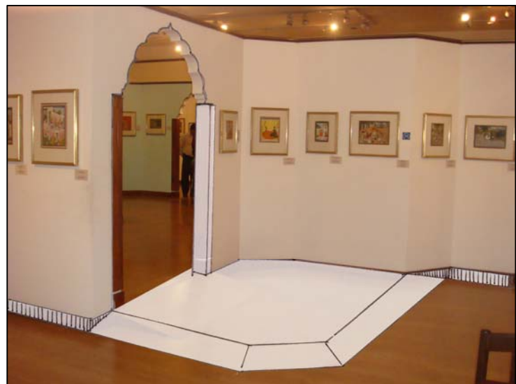
Proposed flared platform with smooth ramp
